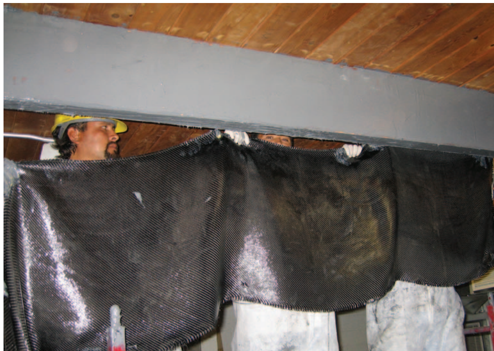
Figure 5: Saturated carbon fabric being applied to the beam surface
