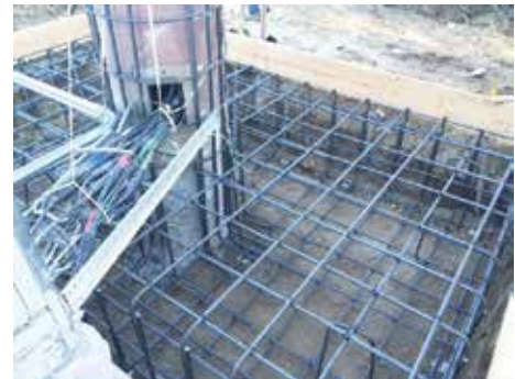
Figure 5. Foundation and the steel dowels at the base of the pole.
