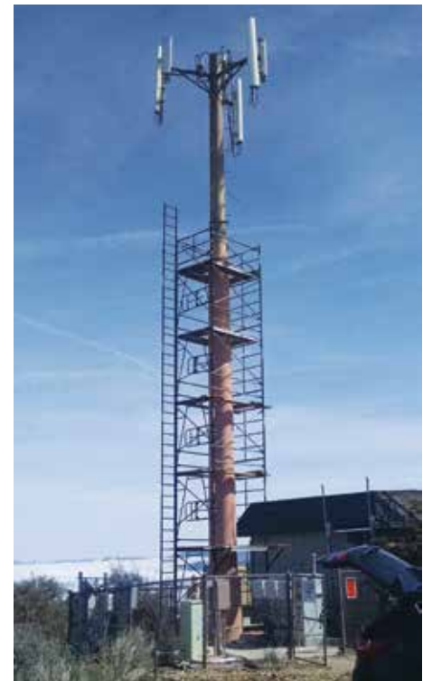
Figure 6. Painted pole at the conclusion of the project.
