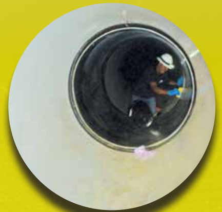
For this pressure pipe repair project, StifPipe™ with an outside diameter of 47 ¼ inch (1200 mm) was constructed with carbon fabric. The pipe was used to slip line the 48 inch (1220 mm) corroded steel pipes with minimal loss of diameter.
