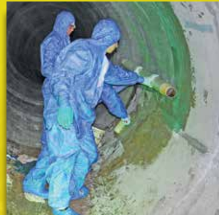
Applying pre-saturated roll of fabric to concrete pipe
