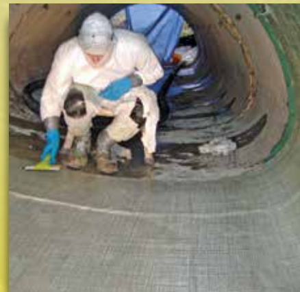
Repair of joints in oval-shaped concrete culvert
