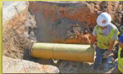
StifPipe™ made with glass fabric was used in the repair of this culvert. The 8 ft (2.4 m) long segments were joined together in the field for slip-lining the deteriorated culvert, and the annular space was grouted.
