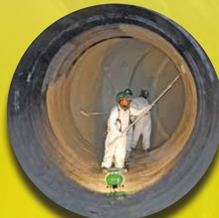
Top coating of CFRP in a curved, large-diameter PCCP
