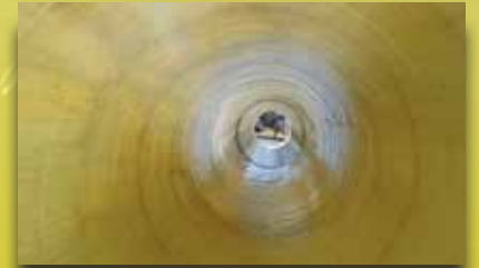
StifPipe™ made with glass fabric was used in the repair of this culvert. The 8 ft (2.4 m) long segments were joined together in the field for slip-lining the deteriorated culvert, and the annular space was grouted.
