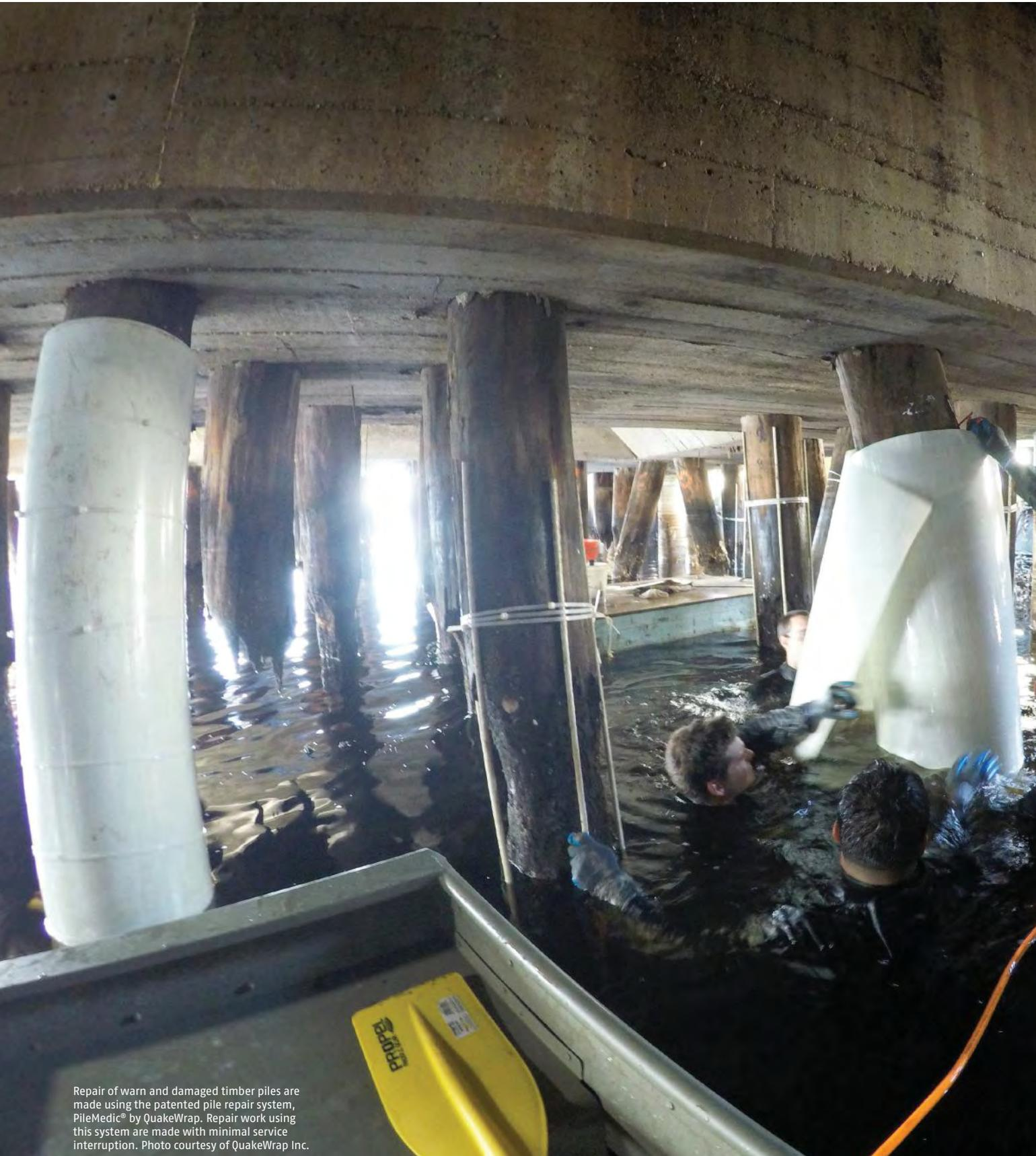
Repair of worn and damaged timber piles are made using the patented pile repair system, PileMedic® by QuakeWrap. Repair work using this system are made with minimal service interruption. Photo courtesy of QuakeWrap Inc.
