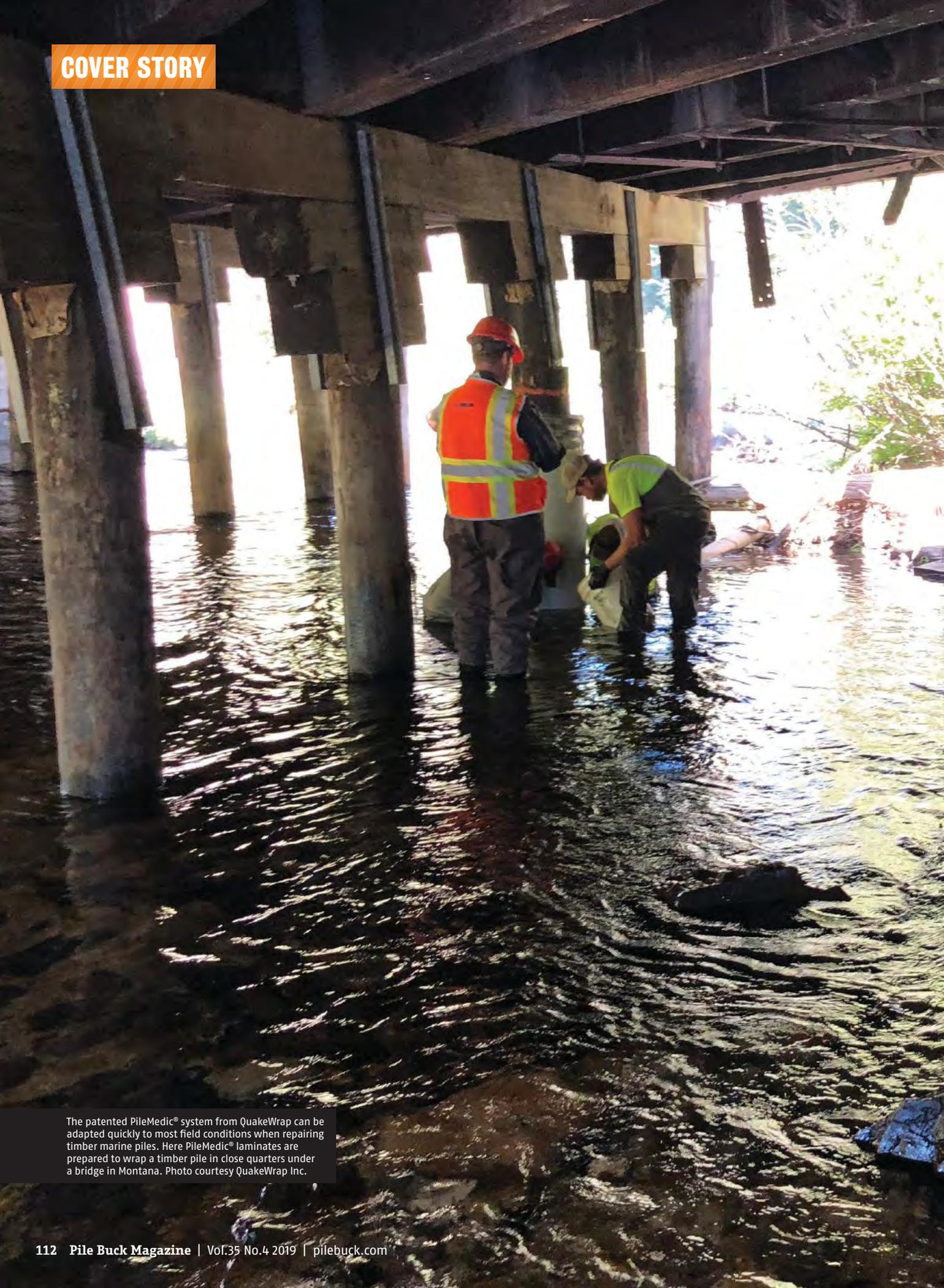
The patented PileMedic® system from QuakeWrap can be adapted quickly to most field conditions when repairing timber marine piles. Here PileMedic® laminates are prepared to wrap a timber pile in close quarters under a bridge in Montana. Photo courtesy QuakeWrap Inc.
