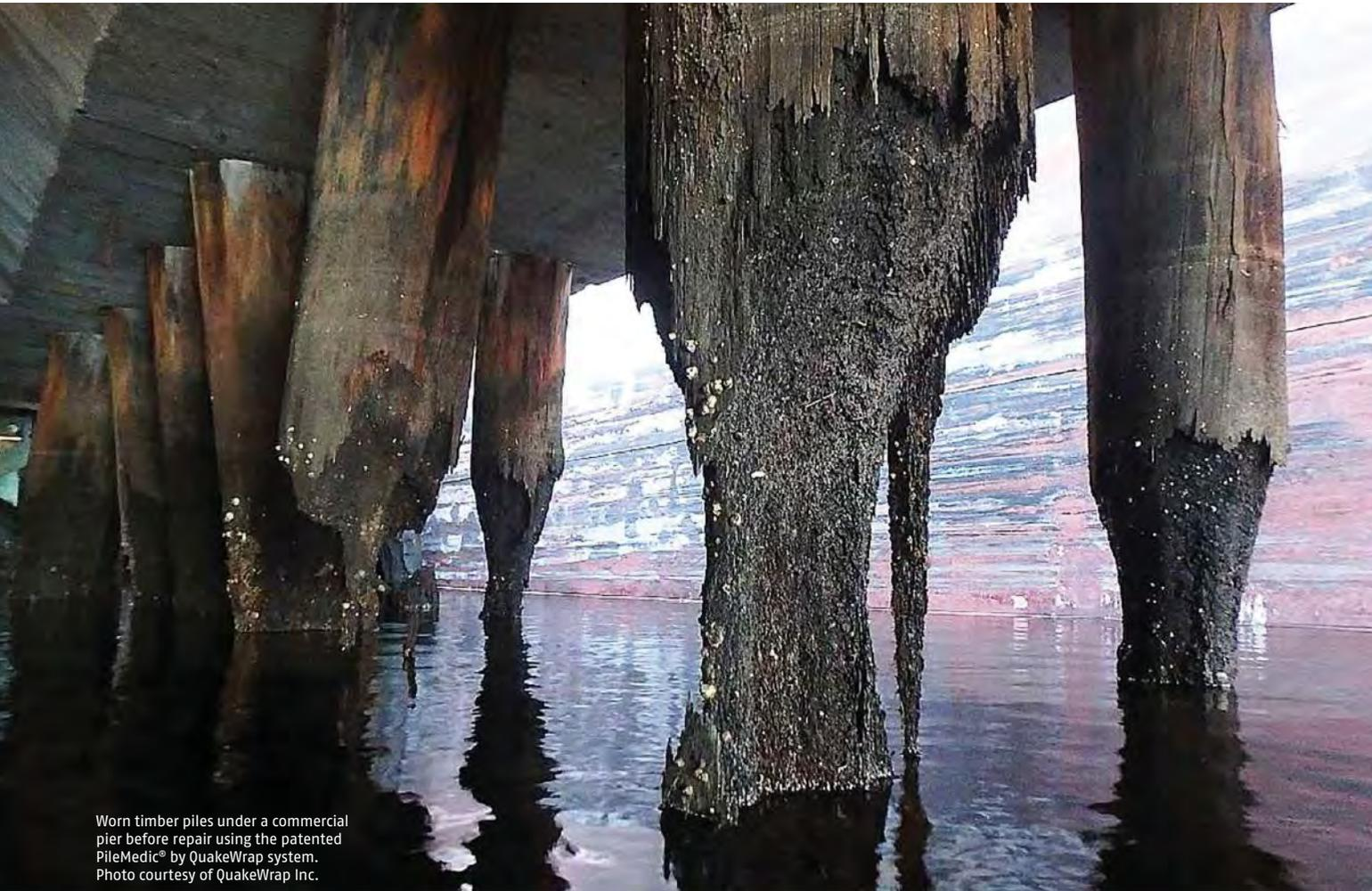
Worn timber piles under a commercial pier before repair using the patented PileMedic® by QuakeWrap system. Photo courtesy of QuakeWrap Inc.
