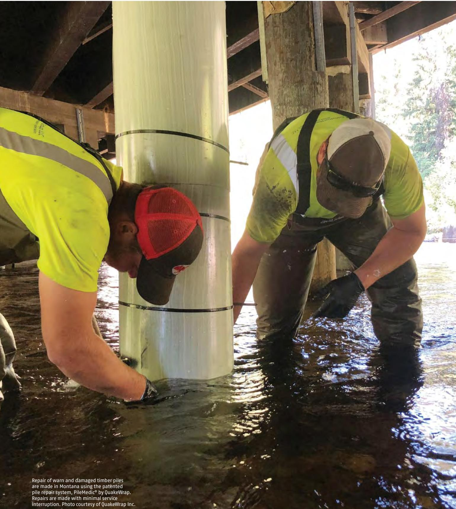
Repair of worn and damaged timber piles are made in Montana using the patented pile repair system, PileMedic® by QuakeWrap. Repairs are made with minimal service interruption. Photo courtesy of QuakeWrap Inc.
