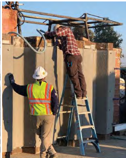
Bair Mock 6: Installed three panel mockup. Photo courtesy QuakeWrap Inc.
