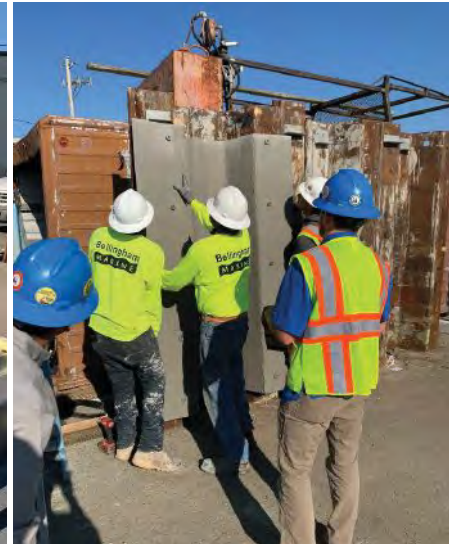
Bair Mock 3: Fit up of first panel. Photo courtesy QuakeWrap Inc.
