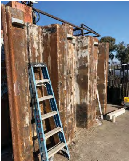
Bair Mock 1: Sheet pile wall matching site conditions. Photo courtesy QuakeWrap Inc.
