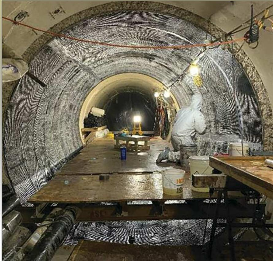
Figure 4. Installation of composite FRP system in a 12-ft tunnel in Minnesota.
