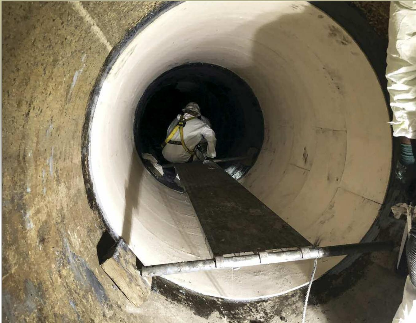
*Figure 3. Installation of StifPipe® with the wet layup method in a 66-inch RCP storm sewer.*
