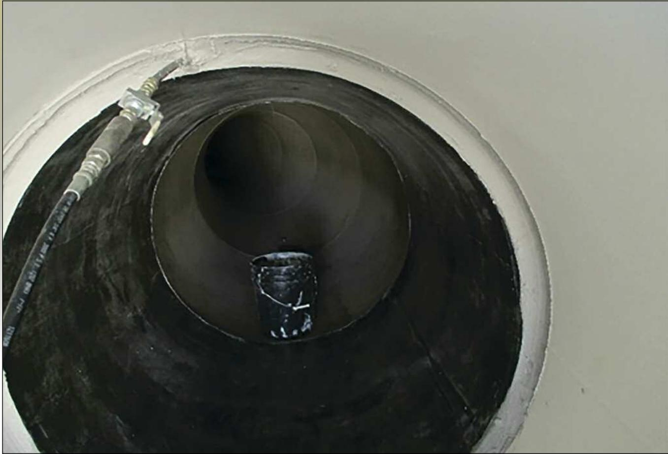
*Figure 2. A post-installation picture from the first application of StifPipe® by sliplining. Note the grout injection port used to fill the annular space.*
