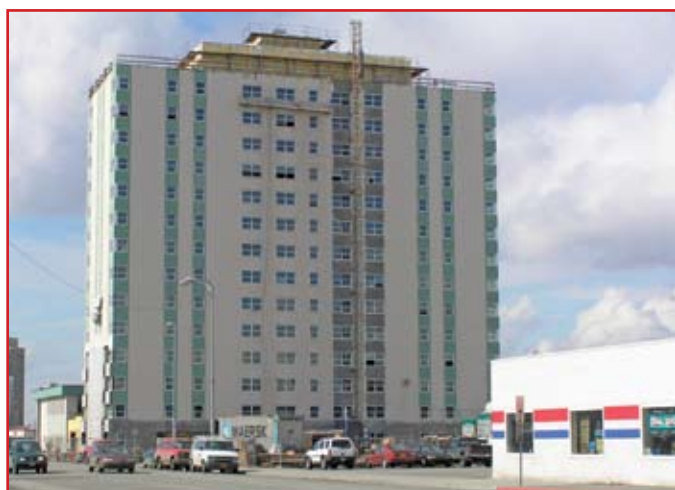
Figure 5: View of nearly-completed and painted building.
