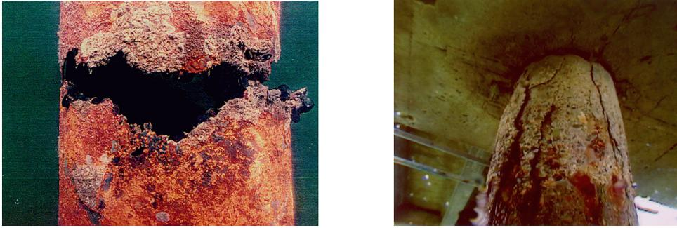
**Figure 1.** Deterioration observed at steel (left) and concrete (right) piles
