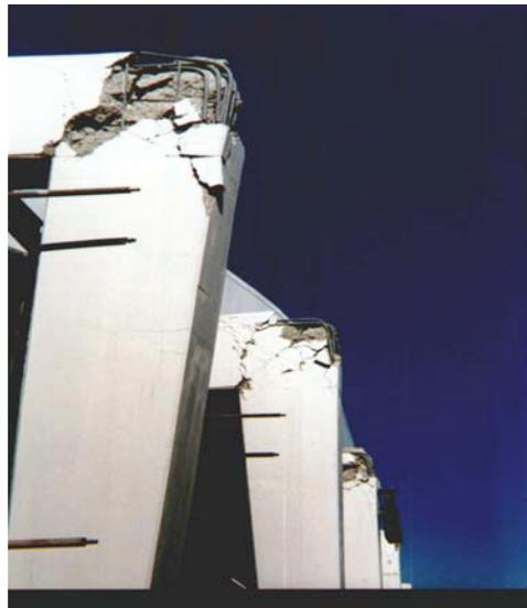
**Figure 1— Local Failure of Beam-Column Connections during Northridge Earthquake, California, 1994. [8]**
