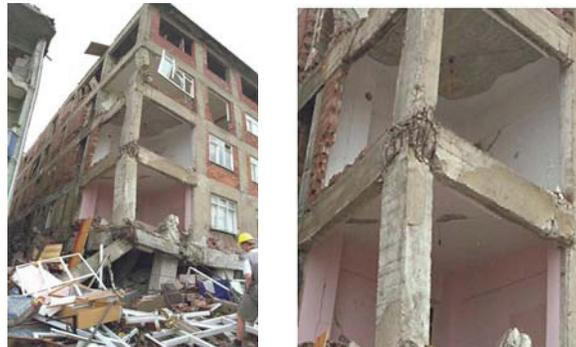
Figure 2— Building Collapse Due To Failure of RC Beam-Column Joints during 1999 Kocaeli Earthquake. [10]
