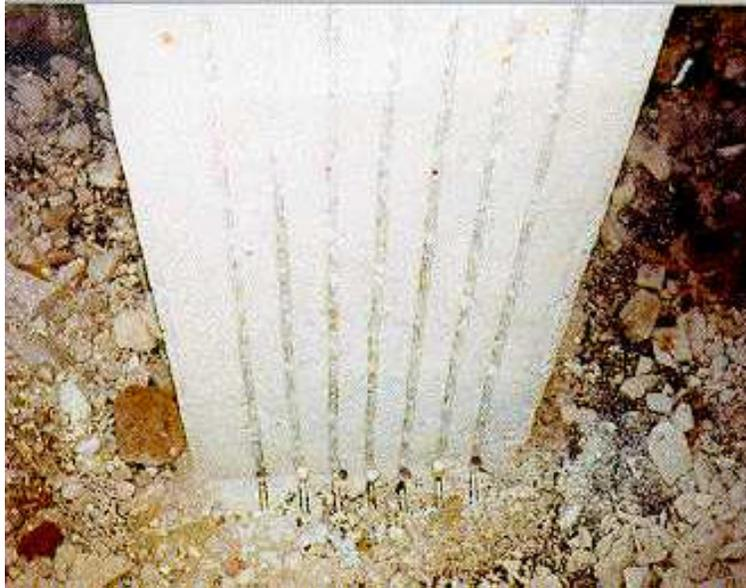
**Figure 1.7. Columns Strengthened with NSM Rods (Alkhrdaji et al., 1999)**
