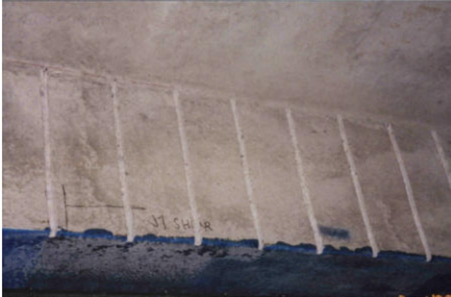
**Figure 1.2. Vertical Grooves for Shear Strengthening with NSM FRP Rods (Hogue et al., 1999)**
