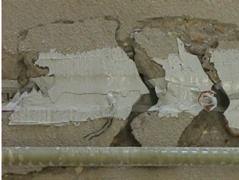
Figure 3.43. Crack Pattern in Specimen G4D24c After Failure
