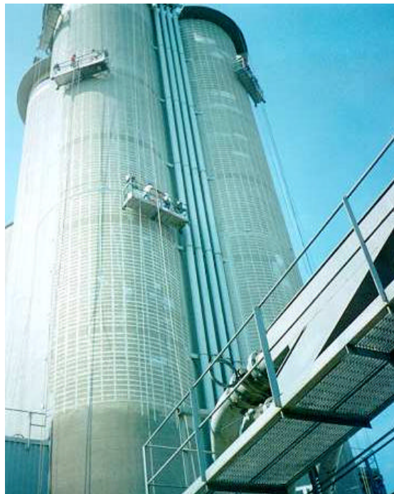
Figure 1.4. Filling of Grooves with Epoxy Paste (Nanni, 1998)
