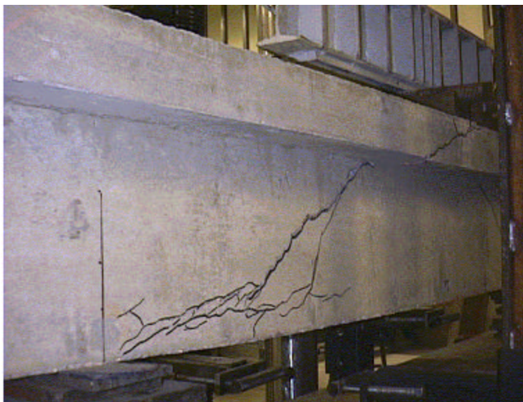
Figure 5.6. Failure of Beam BV
