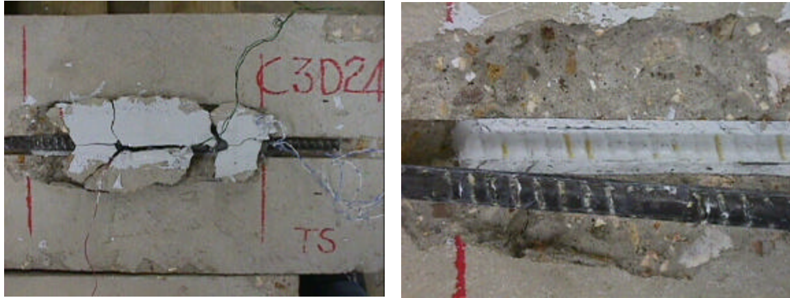
(a) (b) Figure 3.26. Specimen C3D24b After Failure
