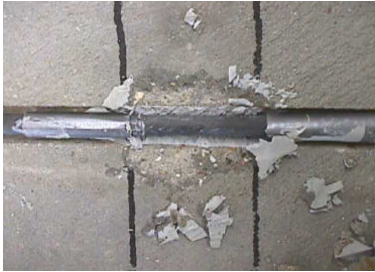
Figure 3.32. Specimen C3S6a After Failure
