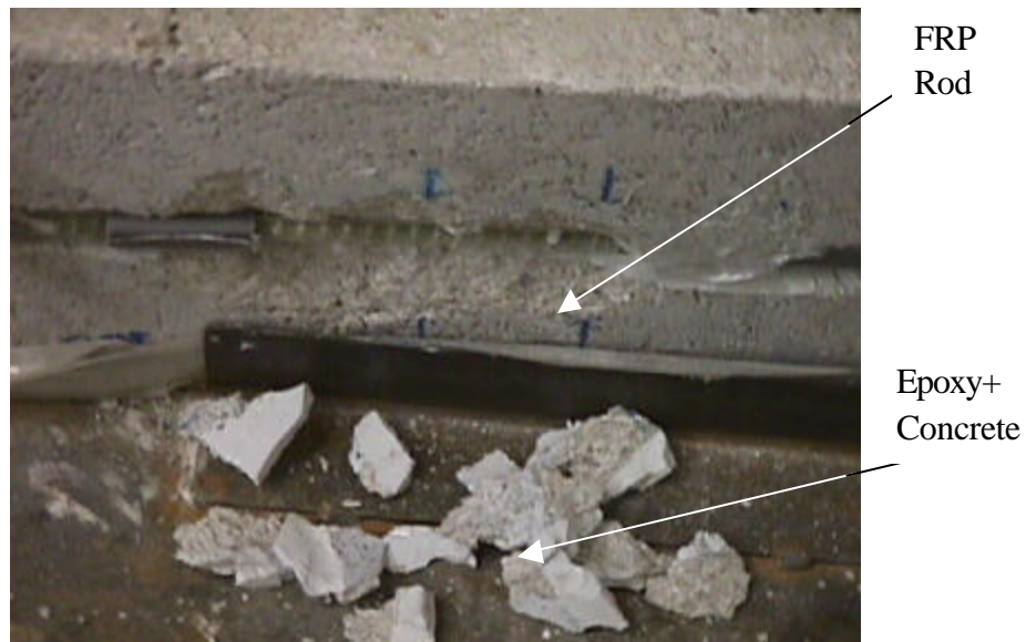
Figure 4.10. Specimen After Splitting Failure
