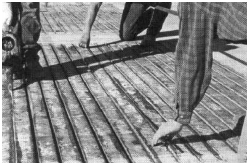
Figure 1.5. Embedding CFRP Rods in the Top Surface of the Deck (Warren, 1998)
