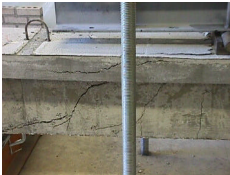
Figure 5.21. Failure of Beam BSV
