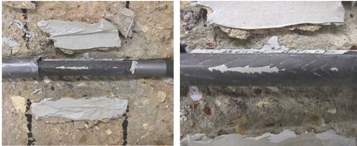
Figure 3.33. Specimen C4S6a After Failure
