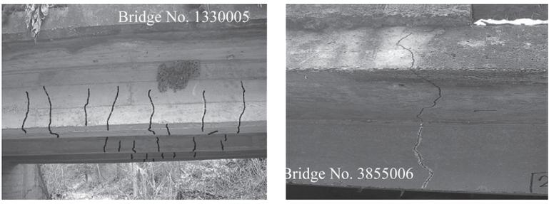
Fig. 4 — Transverse Cracks in Superstructures
