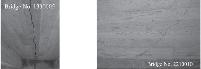
a) Longitudinal Cracks in Decks
