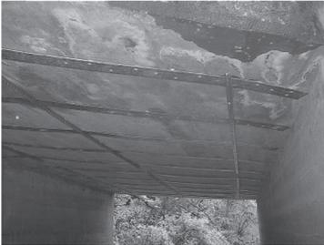
c) Temporary Fixing with Aluminum Angular
