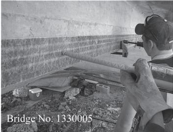
d) Injection of the Epoxy into the Holes
