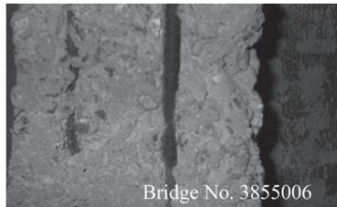
Fig. 3 – Exposed Bars in the Lateral Side of Decks and Girders
