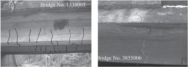
Fig. 4 — Transverse Cracks in Superstructures
