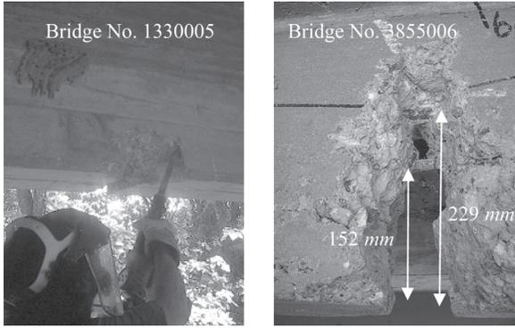
Fig. 6 — Concrete Chipped Off to Find Longitudinal and Shear Reinforcement
