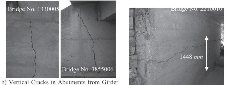
b) Vertical Cracks in Abutments from Girder Edges and Top of Superstructures
