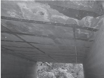
c) Temporary Fixing with Aluminum Angular
