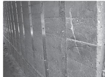
Fig. 11 — Off-System Bridges after Strengthening
