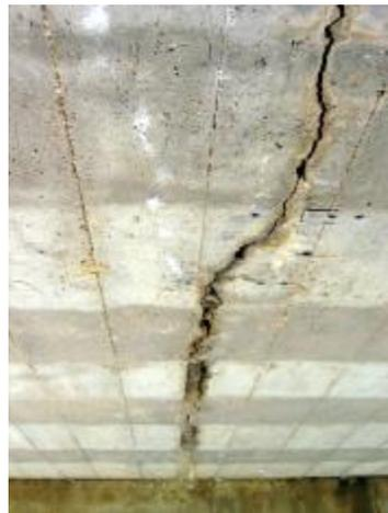
Figure 1-3 - Soffit Slab Longitudinal Crack
