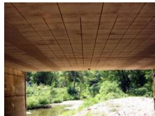
a) Grooves Prepared as per Design Geometry
