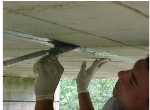
b) Inserting Epoxy Paste into the Groove
