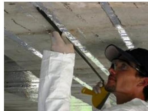
c) Insertion of NSM Bar into the Groove
