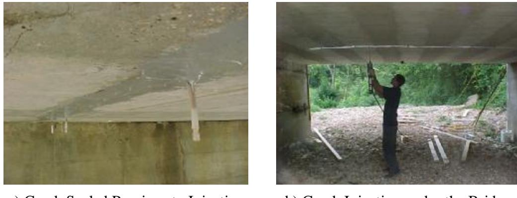
a) Crack Sealed Previous to Injection      b) Crack Injection under the Bridge
