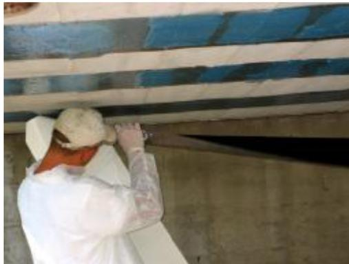
c) Application of CFRP Laminates
