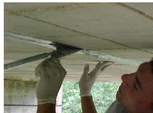
b) Inserting Epoxy Paste into the Groove
