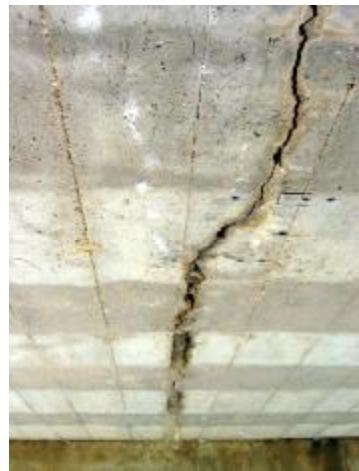
Figure 1-3 - Soffit Slab Longitudinal Crack
