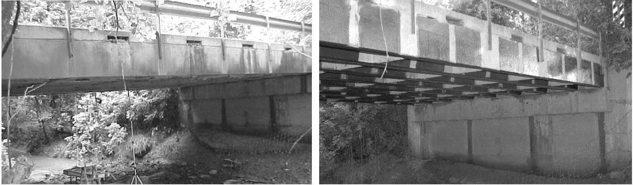
**Figure 4.** CFRP strengthening of Coats Lane Bridge
