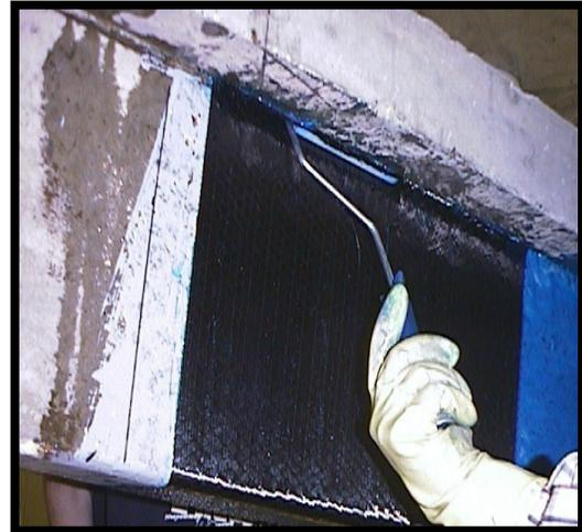
(b) Applying CFRP sheet
