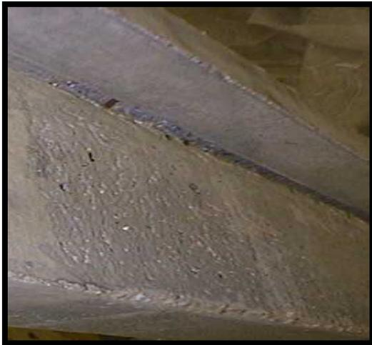
(a) Cutting a groove in the beam flange
