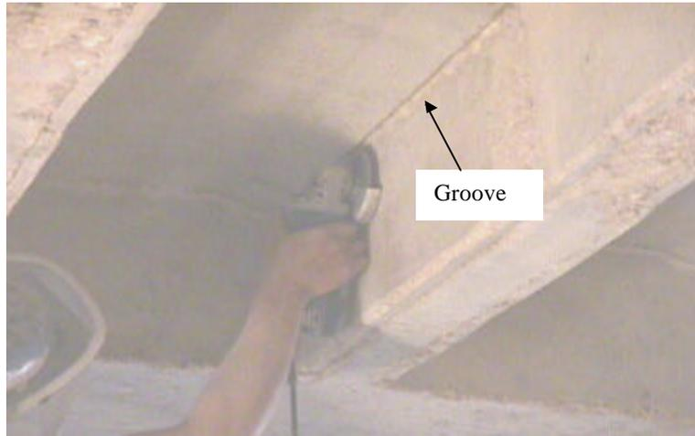
Figure 3.6: Grooves for end anchor
