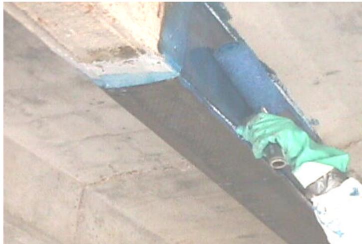
Figure 3.5: Rolling of FRP sheet after the application of saturant
