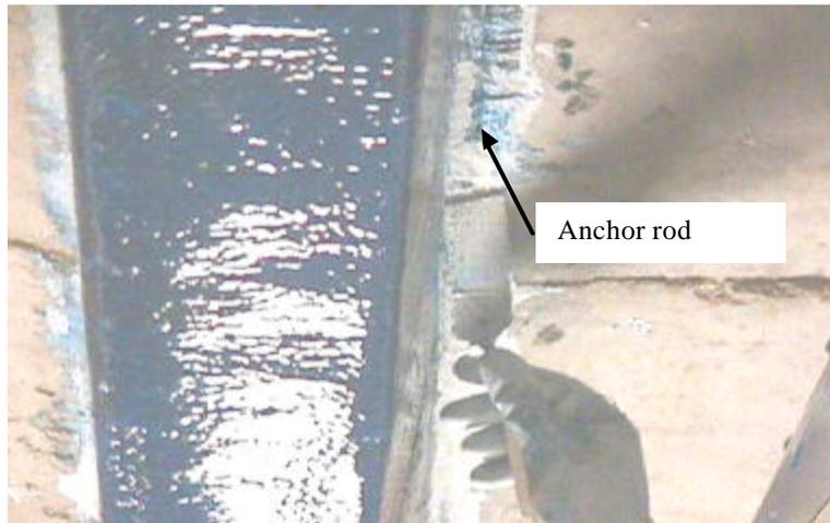
Figure 3.7: Application of epoxy paste to hold the end anchors
