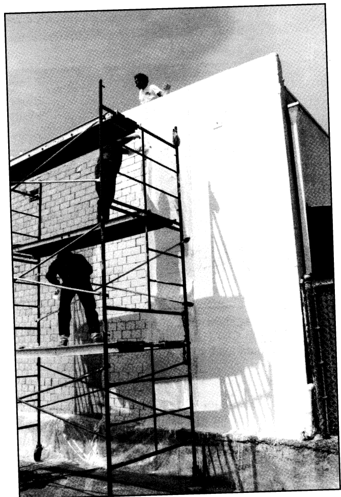
Fig. 12—Application of QuakeWrap ™ to the wall (Photo courtesy of External Reinforcement, Inc.)
