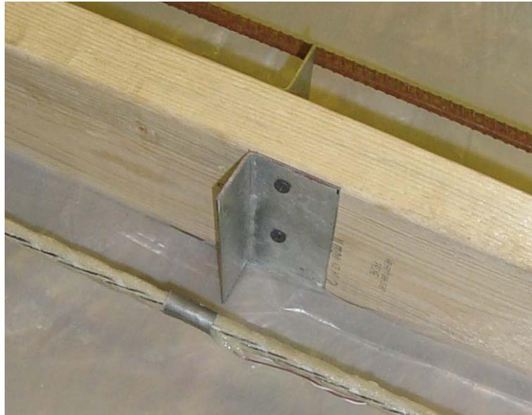
Figure 3.2. Steel Angle Used to Predetermine Crack Location
