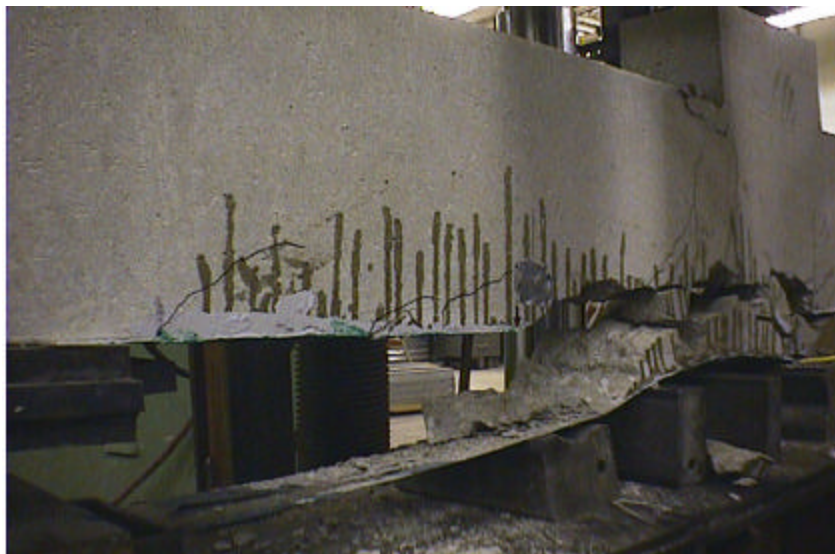
Figure 4.1. Final Failure in Beam A1
