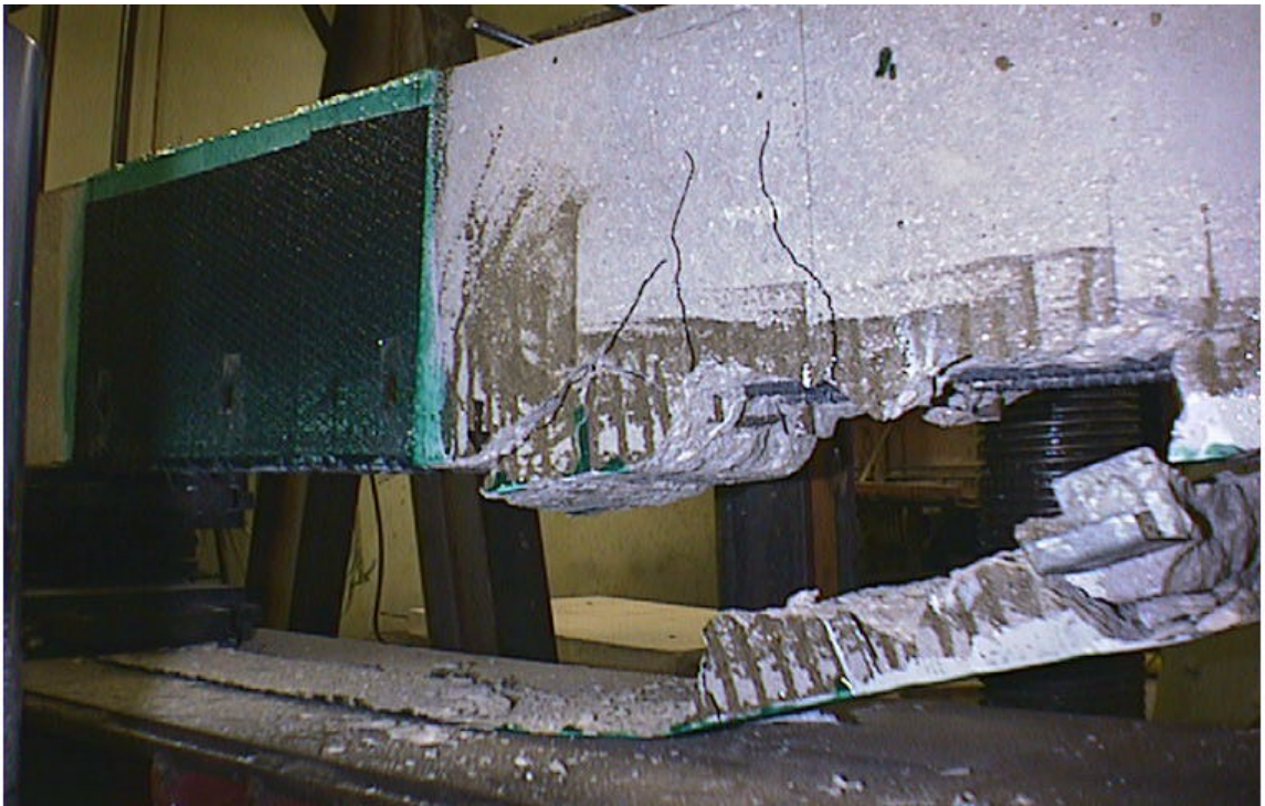
Figure B.4. Failure in Beam A4
