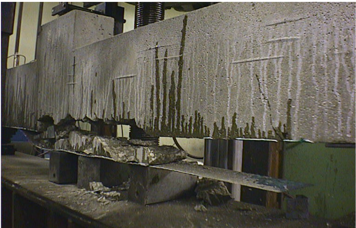
Figure B.8. Failure in Beam C1
