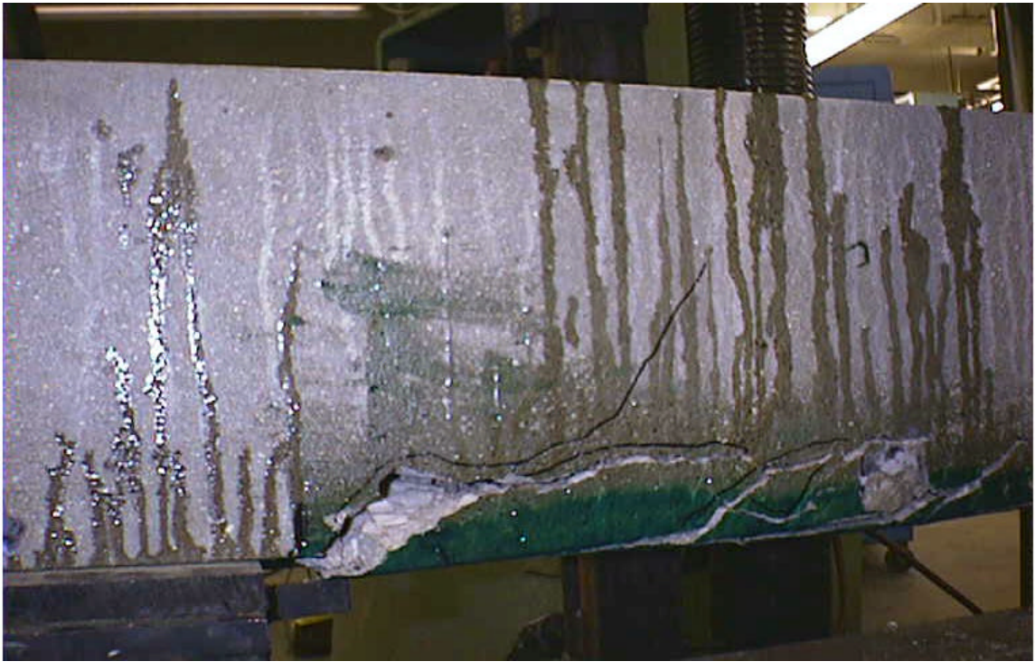
Figure B.3. Failure in Beam A3
