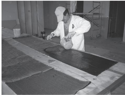
Figure 5 – Saturating of carbon fabrics by hand
