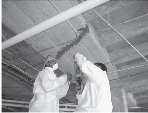
Figure 4 – Crack injection prior to strengthening of beams
