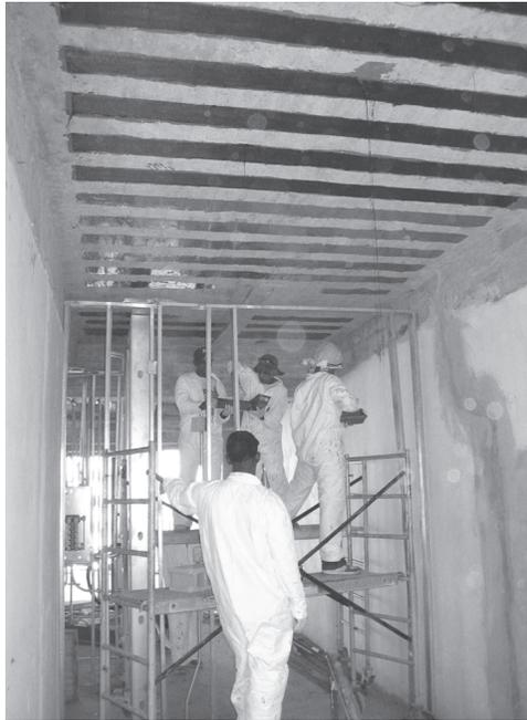
Figure 10 – Strengthening of slab with carbon fabric
