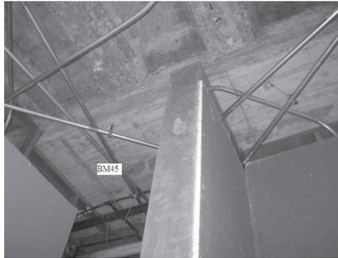
Figure 7 – Partition wall framing crossing the beam axis
