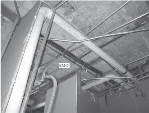
Figure 2 – Utilities limited access to the underside of the beams
