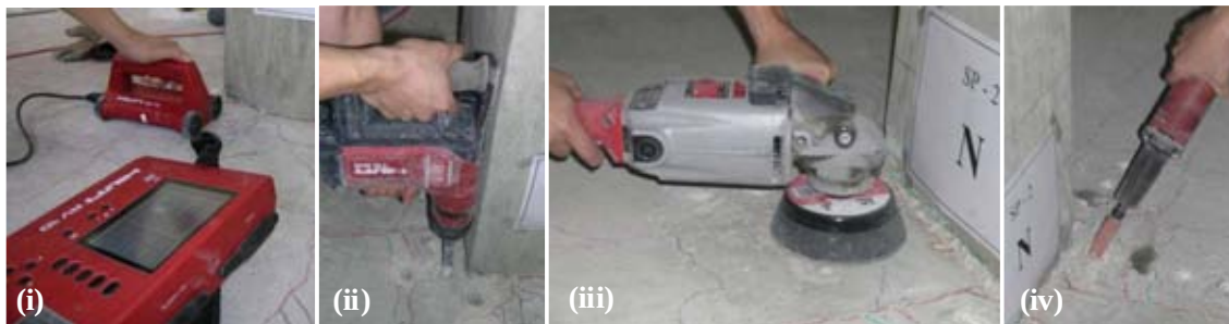
Figure 5. Hole and surface preparation.
