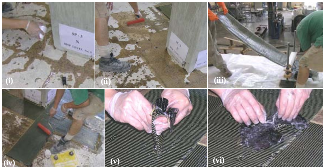
Figure 6. Installation of CFRP sheets and CFRP anchors in SP-3.
