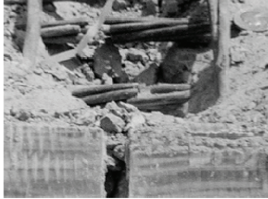
Fig. 13 – Ruptured tendons at location of flexural cracks.
