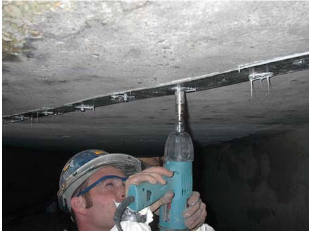
Figure 8. Mechanically Fastened FRP Laminates
