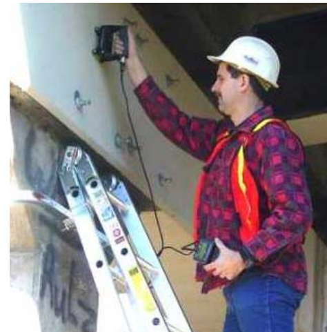
Figure 13. Impact Echo Delamination Testing
