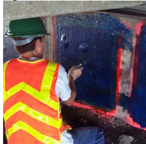
Figure 12. Intentional defects at non-critical locations
