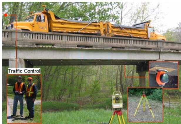
Figure 10. Load Testing – Total Station, Reference Point, Prisms and Traffic Control
