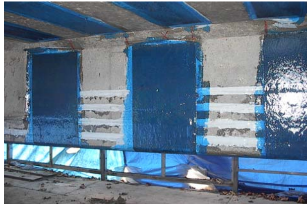
Figure 6. Manual lay-up Laminates and NSM Bars
