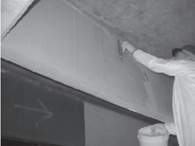
f) Application of Epoxy on U-Wrap
