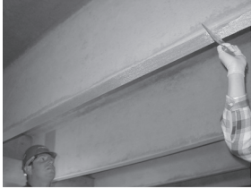
c) Squeezing Out the Resin Excess
