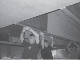
b) Application of Longitudinal Ply
