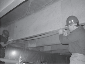
d) Application of Scrim on Longitudinal Ply
