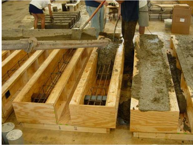
Figure 4.4. Pouring Concrete
