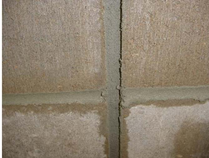
Figure 4.13. Raked Head Joint
