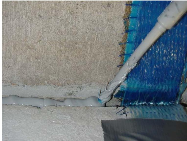
Figure 4.20. Groove Filled with Paste
