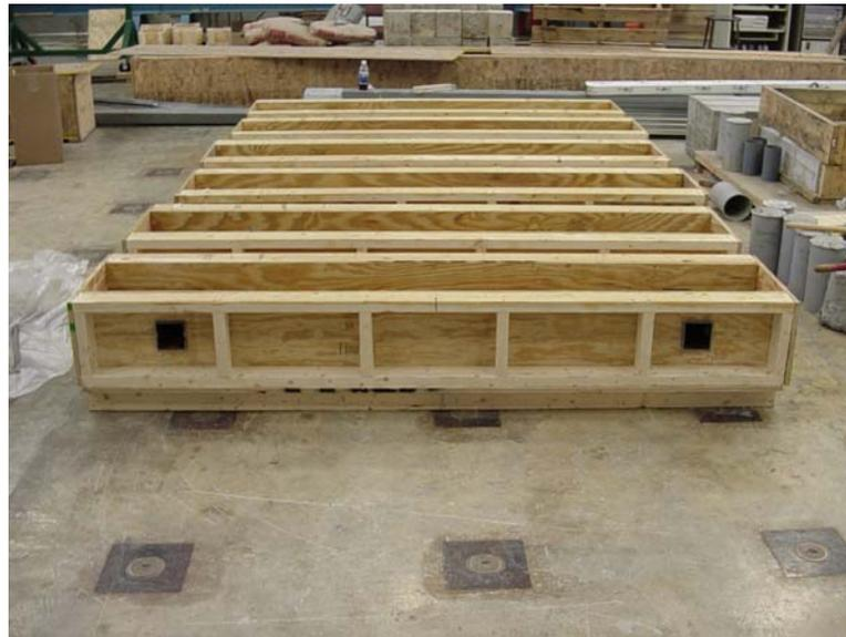
Figure 4.2. Formwork for Boundary Elements
