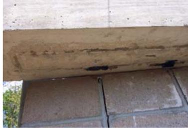
(b) Sliding Failure at Boundary Element
