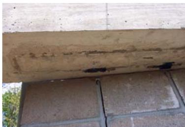
(b) Sliding Failure at Boundary Element
