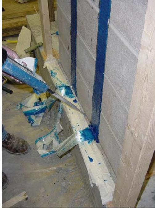
Figure 4.19. Sheet Wrapped in Groove
