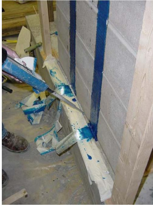
Figure 4.19. Sheet Wrapped in Groove
