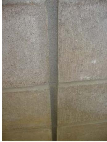
(a) Groove in Vertical Joint
