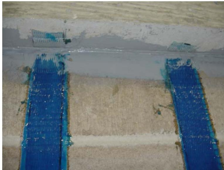
Figure 4.22. Completed GFRP Laminate Anchorage System
