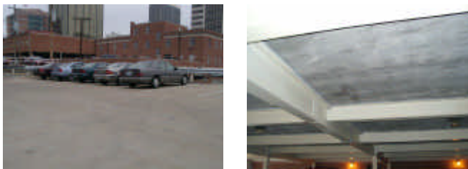
(a) Top Slab View Figure 1 – Parking Garage
