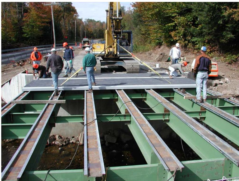
**Figure 12.** Five-Inch Deck Panels Being Installed on the Lewis County, New York, Bridge; October 2001.
