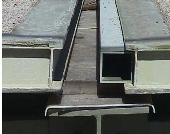
**Figure 4.2 Cross Section of Panel Joint– Jay Street**
