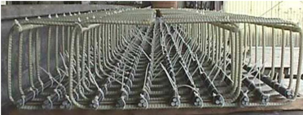
**Figure 3.7 FRP Reinforcement Layout**
