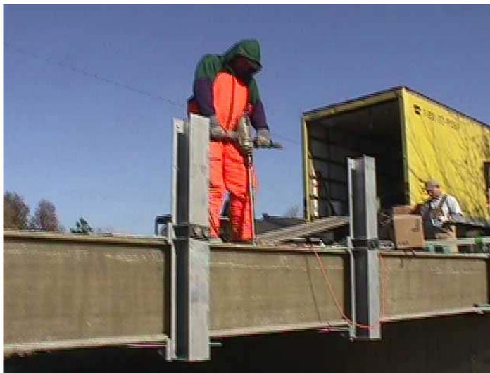
**Figure D.20 Drilling Holes through the Deck to Attach the Guardrails to the Panels – St. Francis Street**
