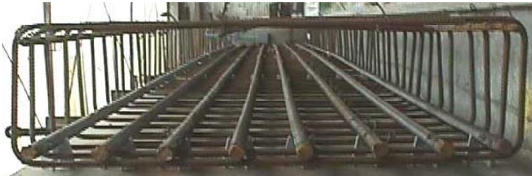
**Figure 6.4 Steel Reinforcement Layout**
