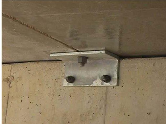
**Figure 4.5 Abutment Connection Detail**
