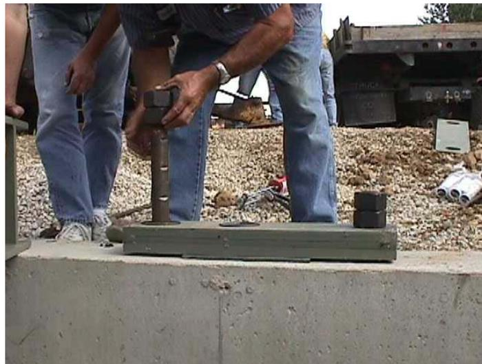
**Figure D.2 Installation of the Bearing Pads, Steel Plates and Anchor Bolts – St. Johns and Jay Street**
