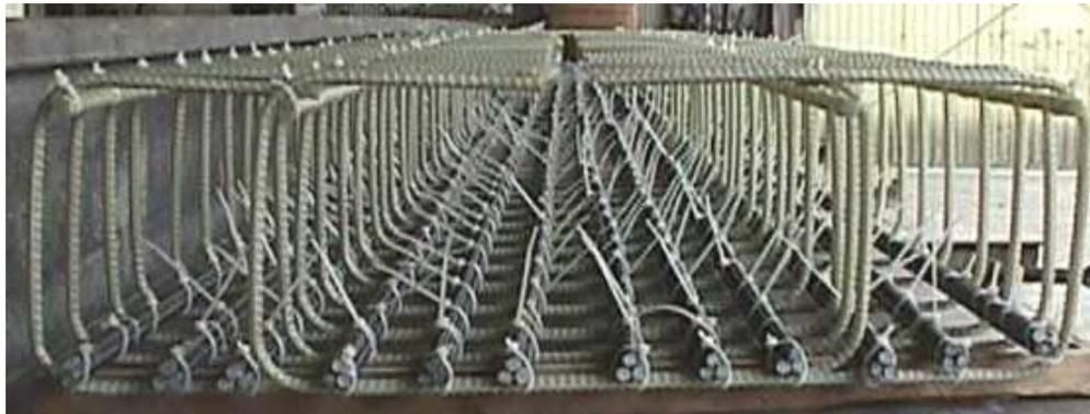
**Figure 3.7 FRP Reinforcement Layout**
