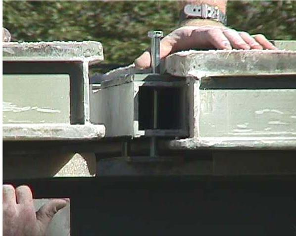
**Figure 4.1 Cross Section of Panel Joint and Clamp Assembly – St. Johns Street**
