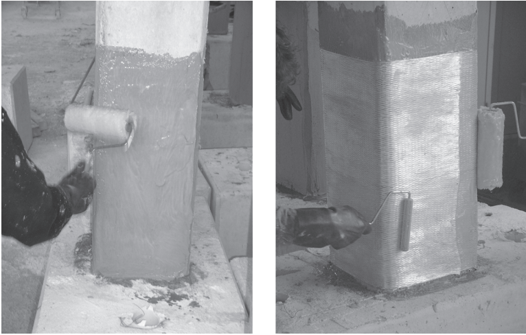
Figure 7 – Installation of GFRP laminates after placement of the steel spikes
