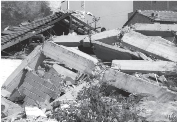
Fig.2—Collapse of the building in the shape of pancake
