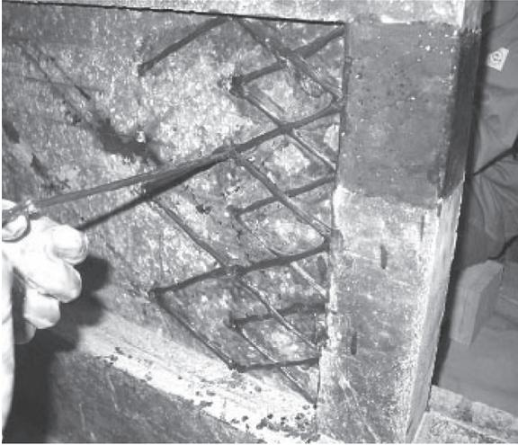
Fig.6—A zigzag sewing path
