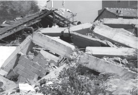
Fig.2—Collapse of the building in the shape of pancake
