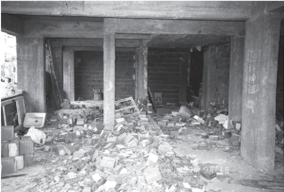
Fig.1—Collapse of the infill-bricks out of the frame
