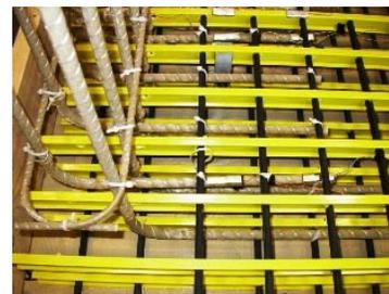
Figure 4 - GFRP reinforcement layout at intermediate post and rail/deck connection
