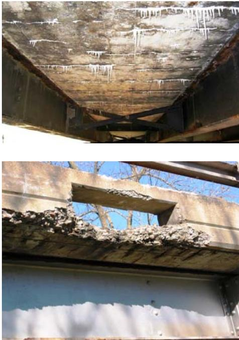
Figure 2 - Degradation of deck, girder and safety appurtenance of Bridge 148, Greene County, MO
