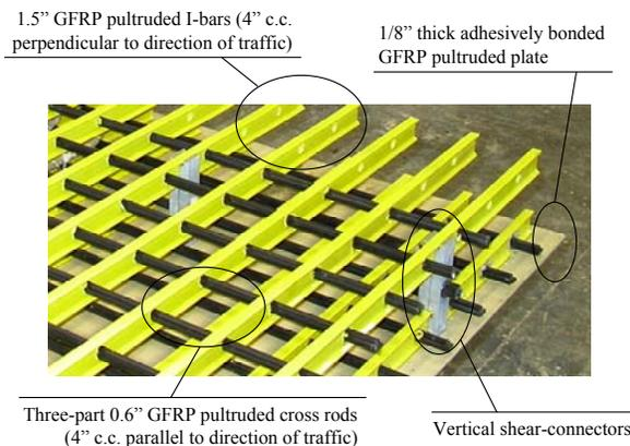
Figure 3 - GFRP SIP deck reinforcement panel
