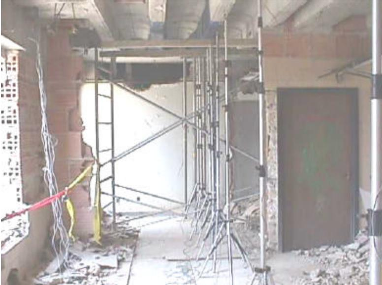
Figure A.10: Typical instrumentation setup below the test member
