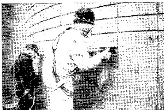
Fig. 4-4: Saw-cutting grooves for NSM reinforcement
