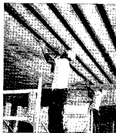
Fig. 4-3: Installing FRP plates on a concrete slab
