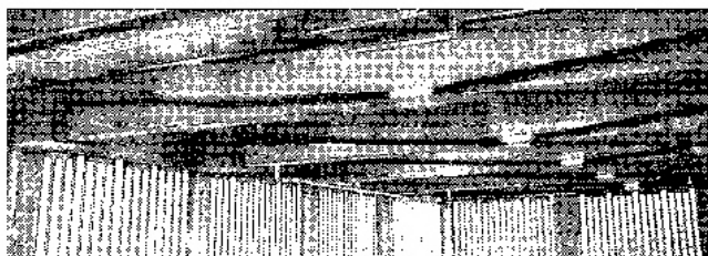
Fig. 5-7: Externally post-tensioned concrete beams
