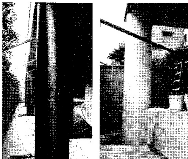
Fig. 4-17: Column confinement using CFRP fabric before and after the acrylic-based protective coating was applied
