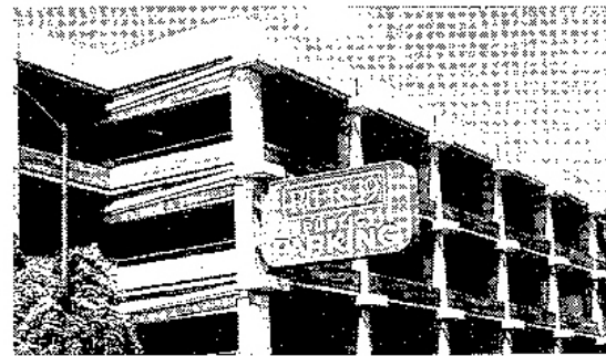
Fig. 5-4: External PT system encased in concrete
