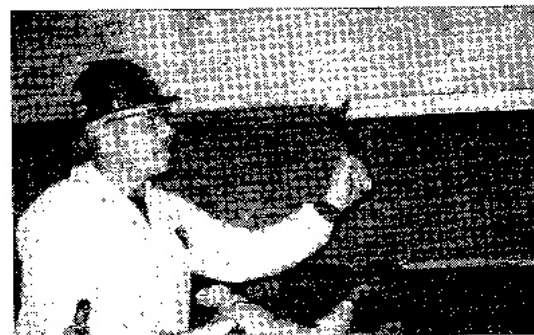
Fig. 4-7: SRP reinforcement applied with cementitious grout for precast joist upgrade
