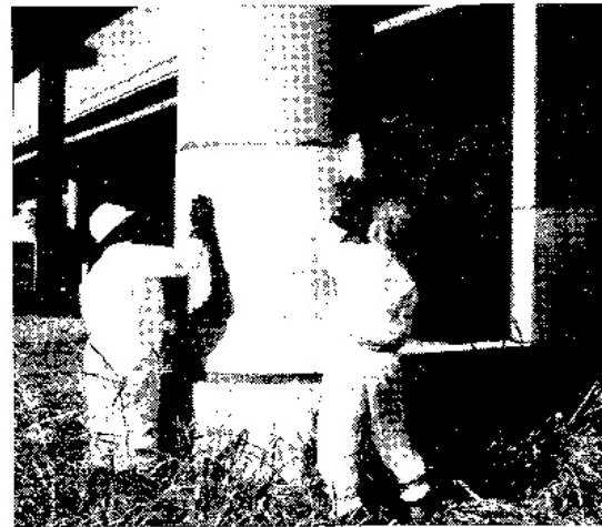
Fig. 4-14: Seismic strengthening of bridge piers with GFRP fabrics
