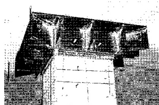
Fig. 6-8: Support extension at top of column to increase punching shear capacity
