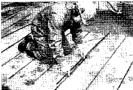
Fig. 4-13: Negative moment reinforcement of slab with surface mounted CFRP bars
