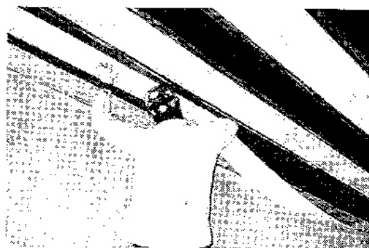
Fig. 4-2: Installing FRP fabric system on a slab soffit
