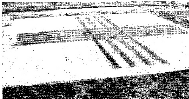
Fig. 4-11: Slab strengthening with CFRP plates for negative moment reinforcement
