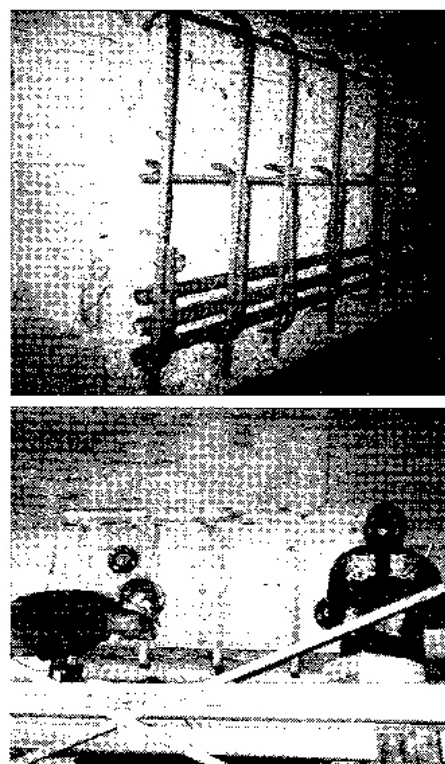
Fig. 3-1: Beam enlargement preparation and form and pump technique
