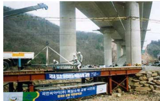
Figure 29. Installation of composite deck
