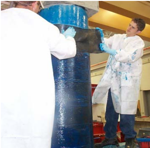
Figure 2. FRP Wrapping on a Column
