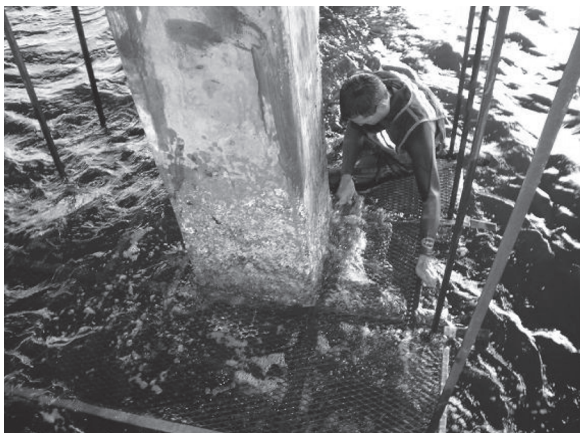
Figure 10 — Scaffolding System, Gandy Bridge, Tampa
