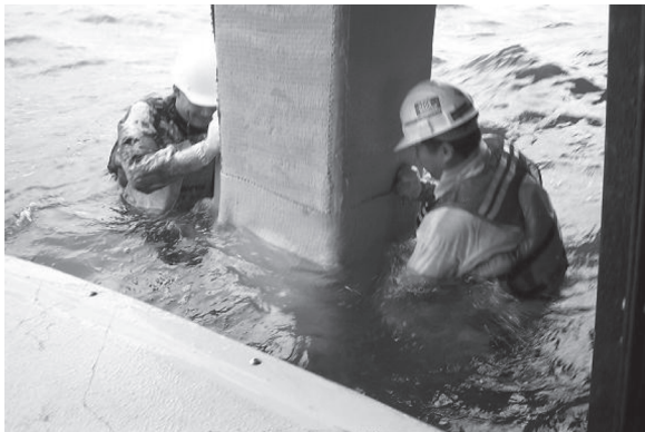
Figure 6 — Underwater Wrapping, Friendship Trails Bridge, Tampa
