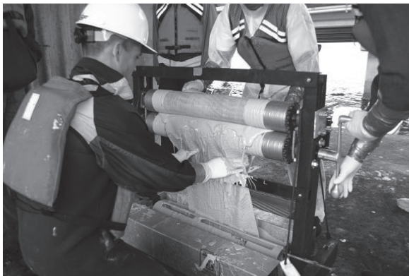
Figure 7 — On-Site Saturation, Friendship Trails Bridge, Tampa
