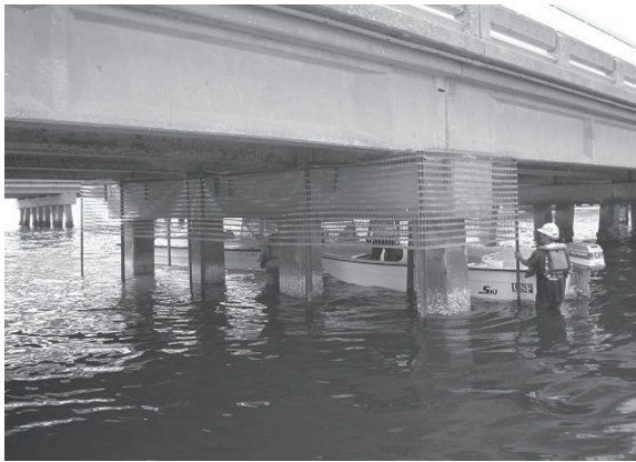
Figure 4 — Scaffolding System, Friendship Trails Bridge, Tampa, FL
