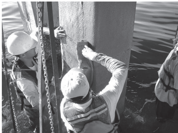
Figure 11 — Underwater Wrapping, Gandy Bridge, Tampa
