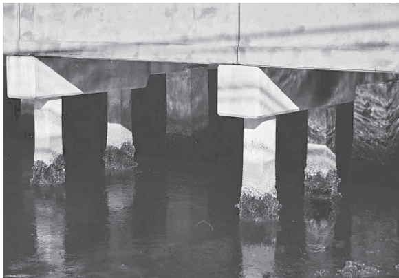
Figure 2 — Marine Growth, Allen Creek Bridge, Clearwater
