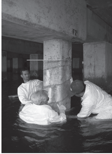
Figure 3 — Underwater Wrapping, Allen Creek Bridge, Clearwater
