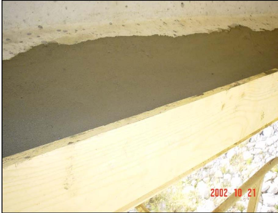
**Figure A-6-** *Patch material for concrete repair*
