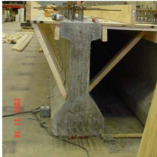
**Figure B-17-** *Formwork preparation*
