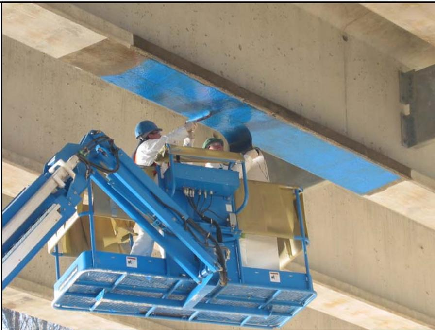
**Figure A-15-** *Application of second layer of saturant*
