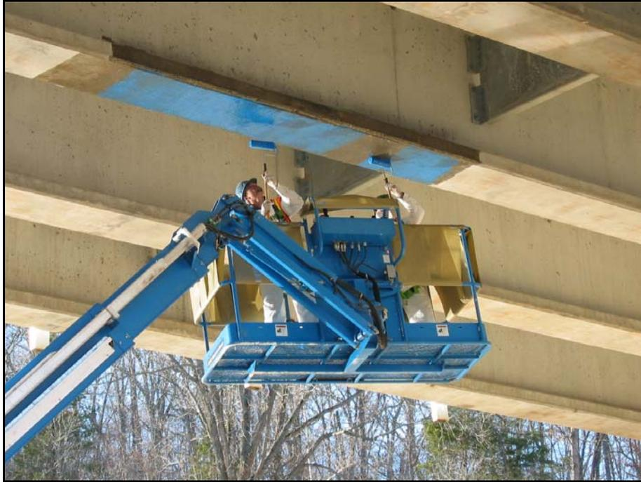
**Figure A-12-** *Application of first layer of saturant*
