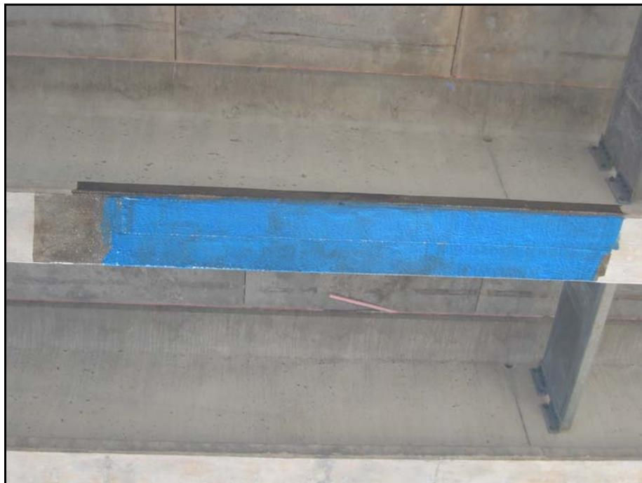
**Figure A-17-** *First ply of CFRP application completed*
