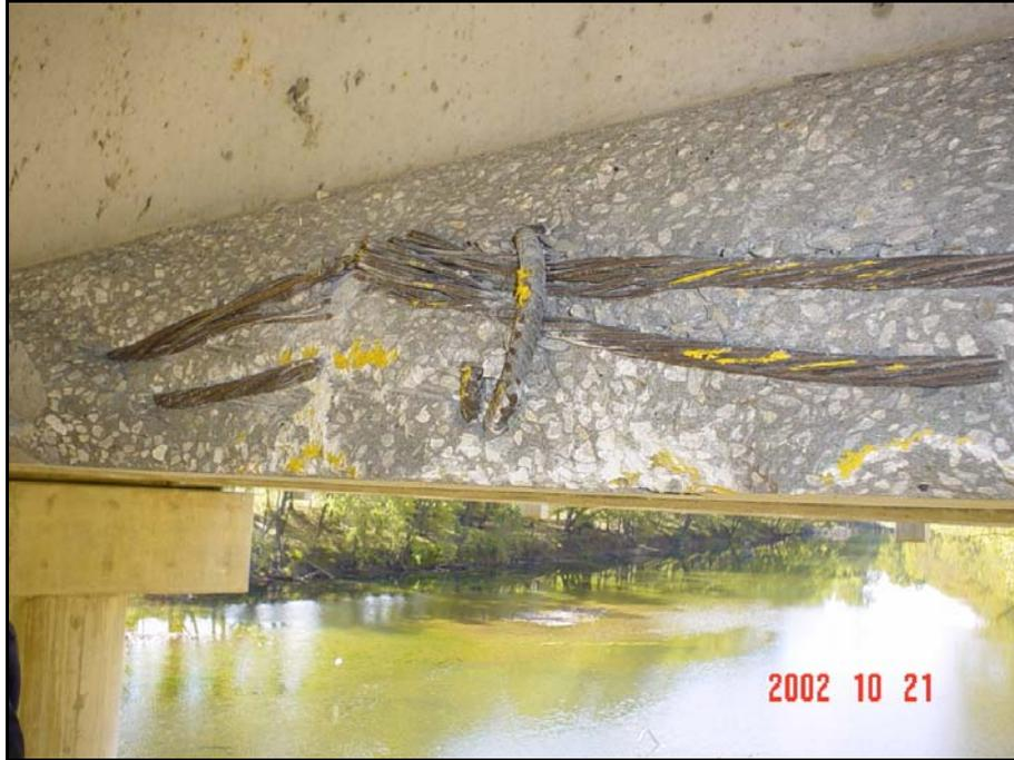
**Figure A-4-** *Spalled concrete and two tendons fractured*
