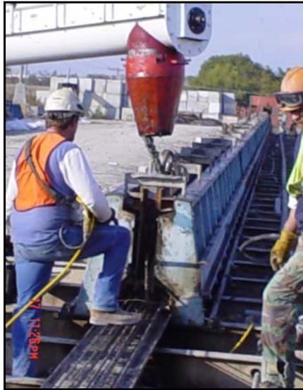
**Figure B-13- Girder casting**
