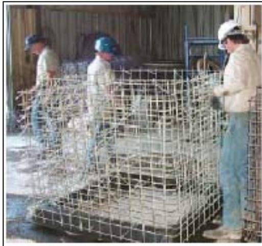
Figure I-8-2- *GFRP cage*
