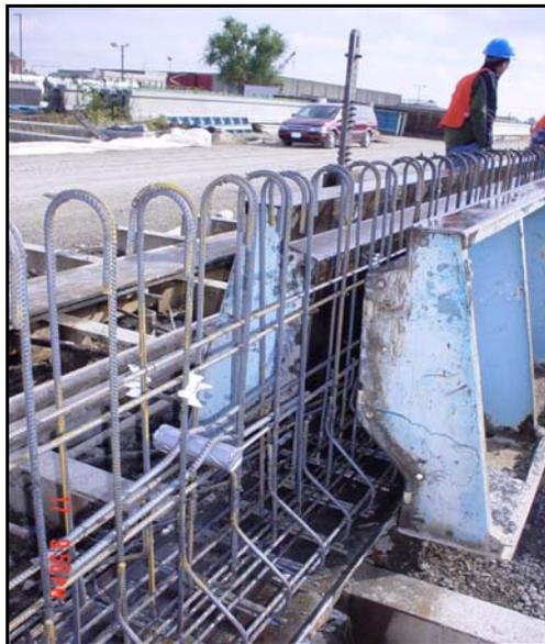
**Figure B-12- *Formworks installation***
