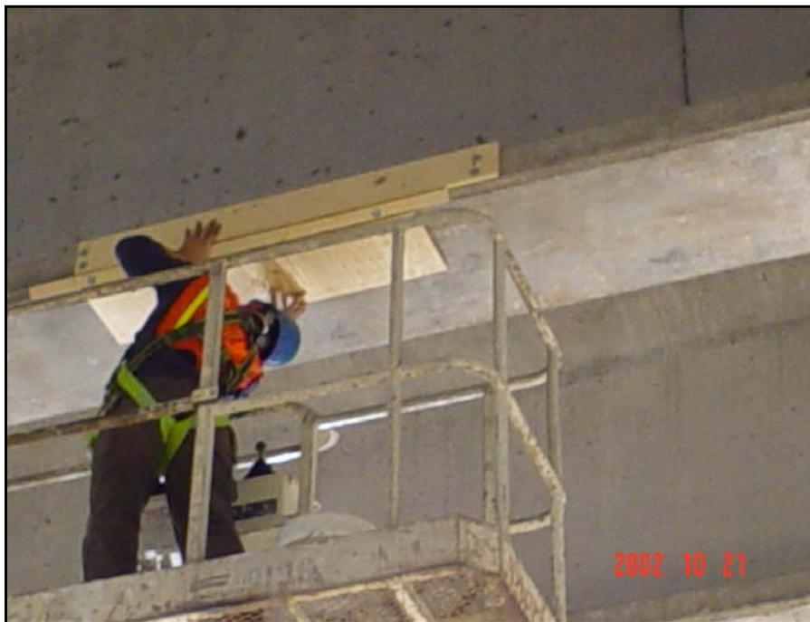
**Figure A-5-** *Formwork application to restore damaged area*
