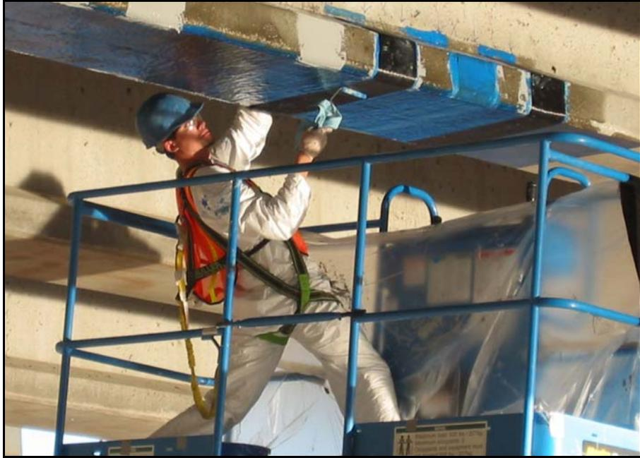
**Figure A-20-** *U wrap installation: strips application*
