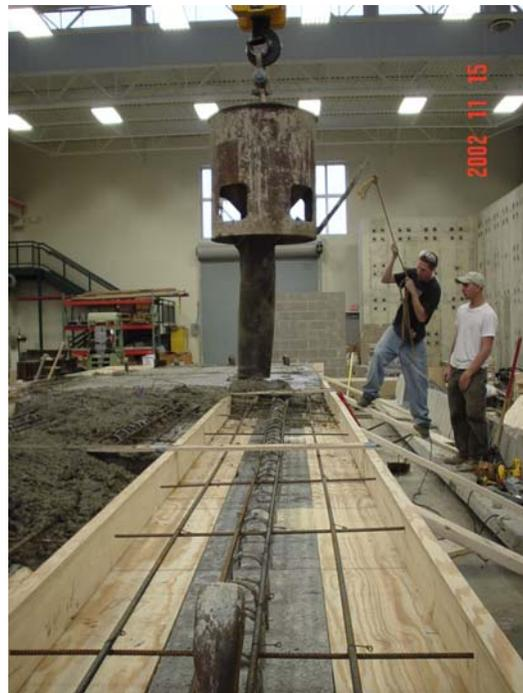
**Figure B-19-** *Deck casting*
