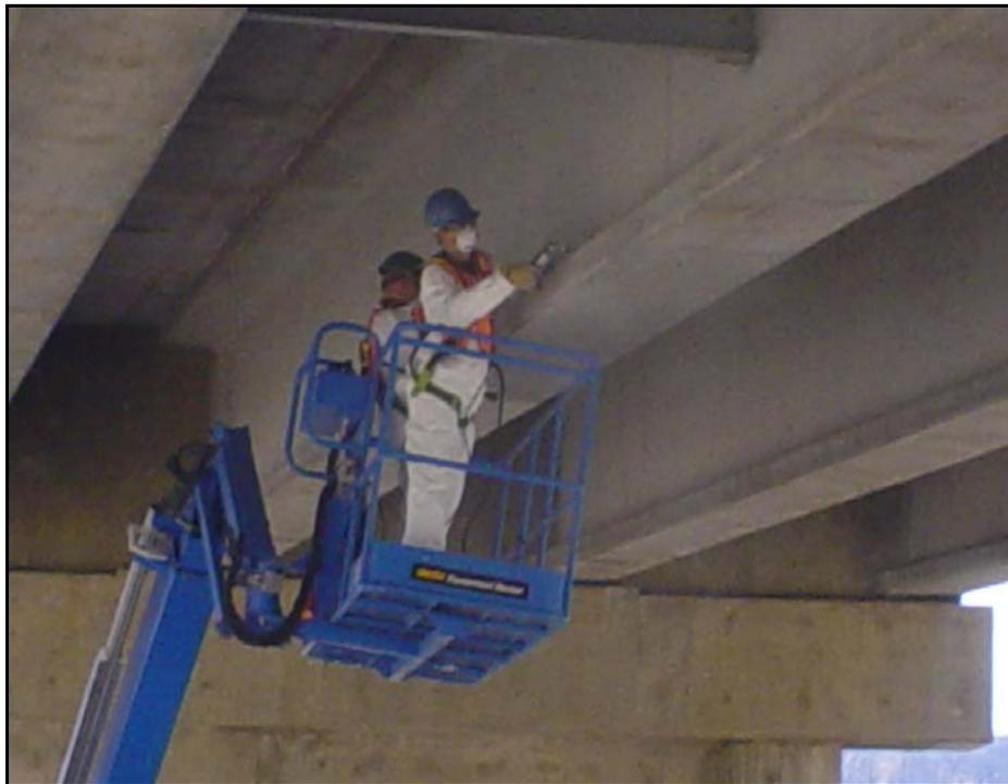
**Figure A-7-** *Bottom edges of the girder rounded for proper installation*
