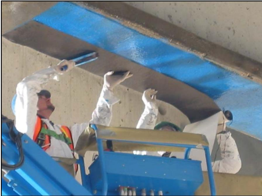
**Figure A-14-** *Application of FRP laminate*
