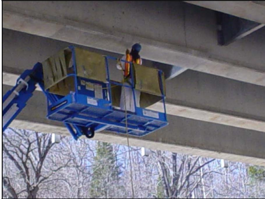
**Figure A-8-** *Sandblasting of the repaired area*
