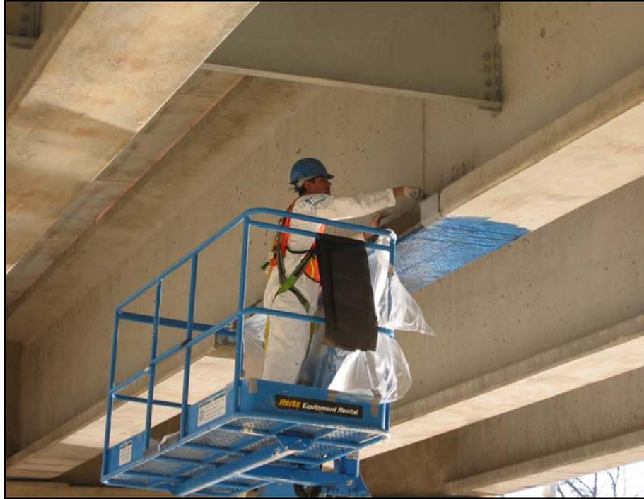
**Figure A-18-** *U-wrap installation*
