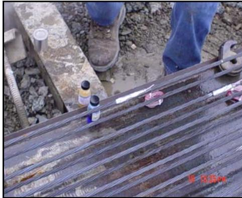
**Figure B-7-** *Strain gage protection*
