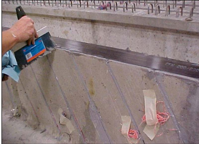
**Figure IV-2-2 - Removal of excess resin**
