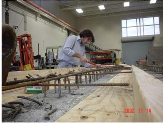
**Figure B-18-** *Steel reinforcement installation*
