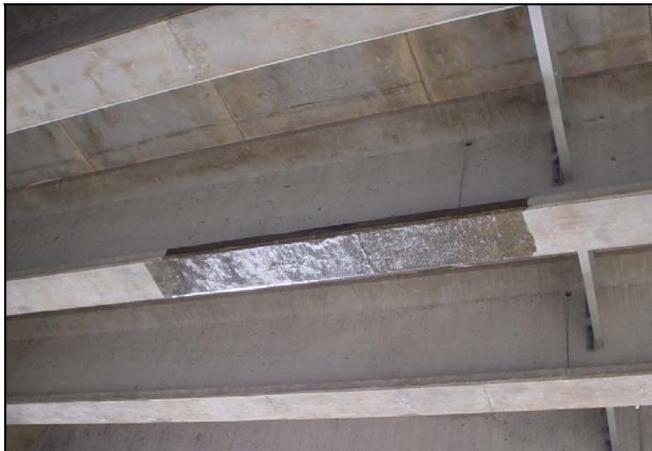
**Figure A-11-** *Application of primer completed*
