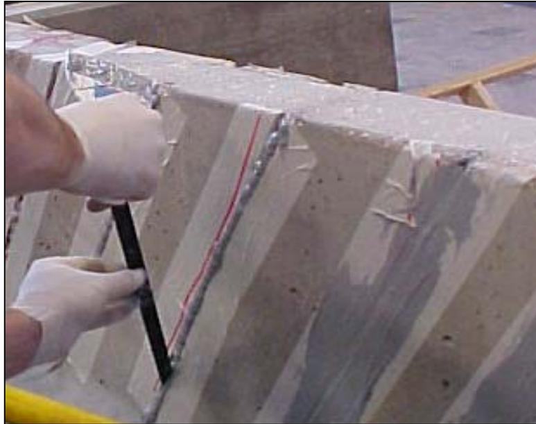
**Figure IV-2-3** - *Installation of rectangular CFRP bar for shear strengthening*
