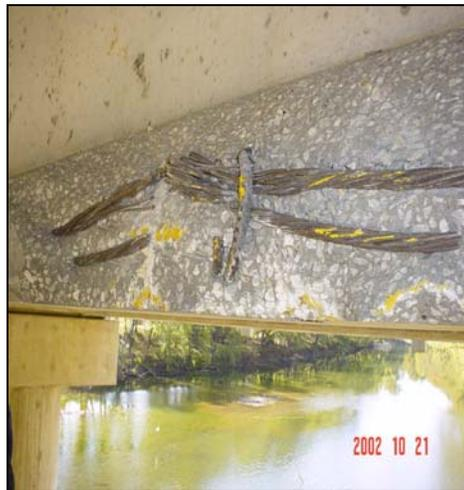
**Figure II-2-3– Damaged Area in the girder**
