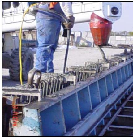
**Figure B-14- Girder Concrete vibration**
