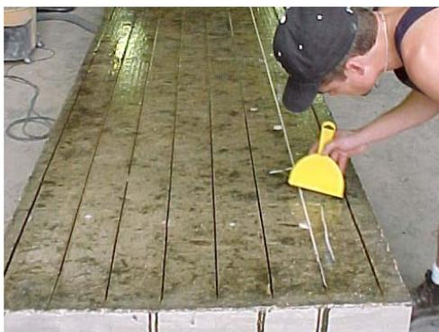
(c) Press down the CFRP bar
