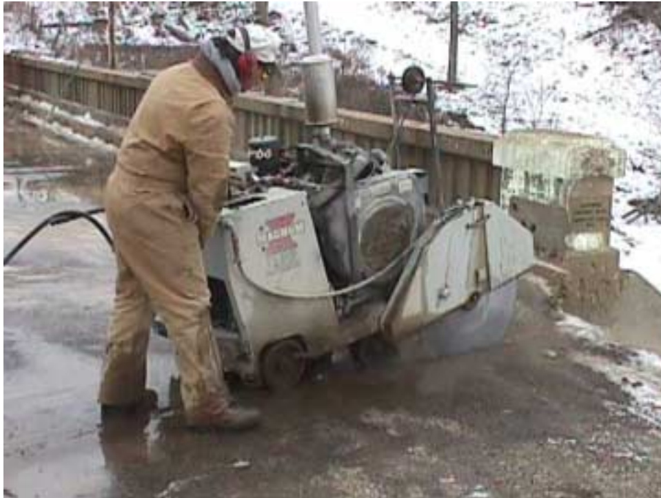
Figure 4.15. Cutting bridge deck joints.
