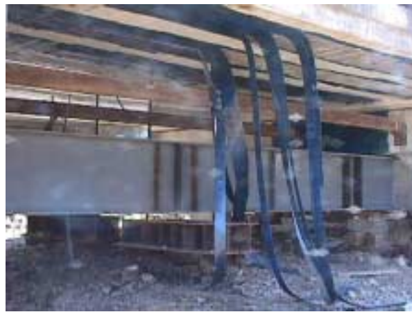
(b) Peeling of CFRP sheets
