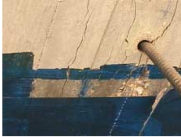
(a) Rupture of CFRP at formlines
