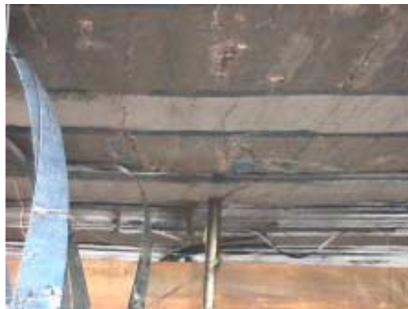
(c) Close up showing peeling of CFRP sheets
