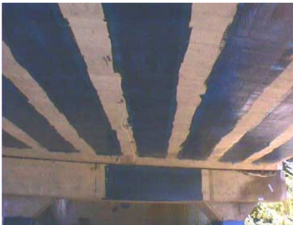
Figure 3.10. Deck 2 after strengthening with CFRP sheets.
