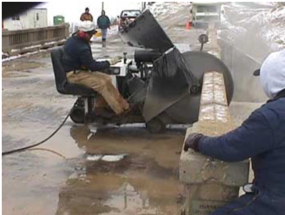
Figure 4.16. Cutting bridge parapet walls.
