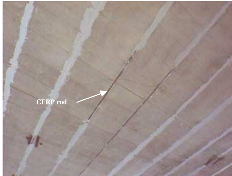
Figure 3.7. FRP rods before applying the second layer of paste.
