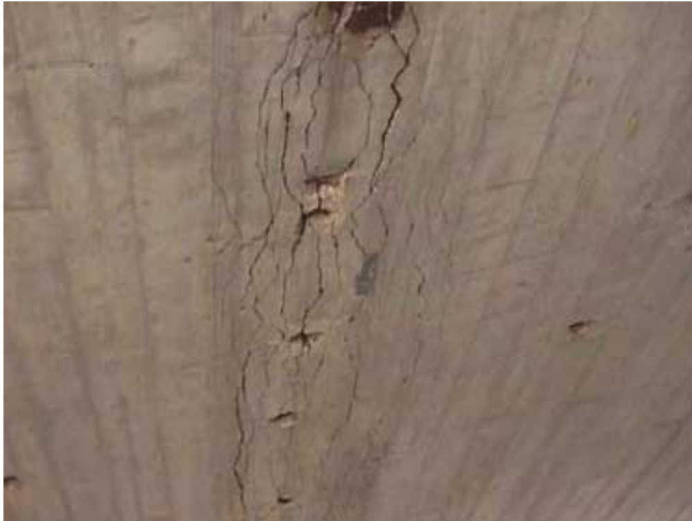
(a) Cracks on the deck soffit testing
