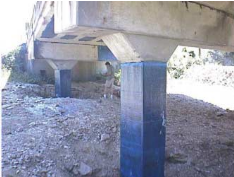
Figure 2.13. Photo showing the bridge after strengthening.
