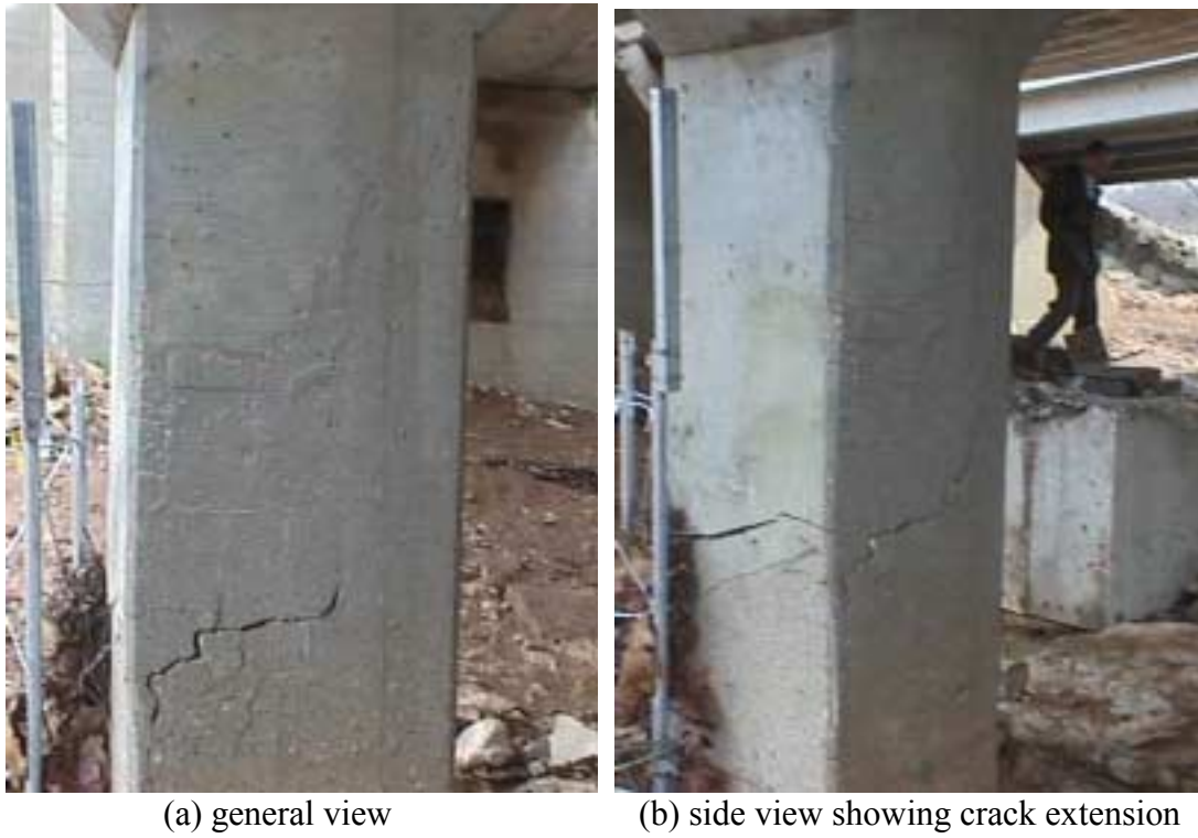
Figure 4.7. Crack on Column B2P1.
