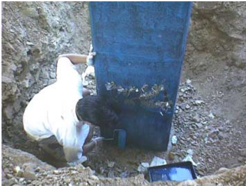
Figure 2.11. Applying the bottom lift of the jacket.
