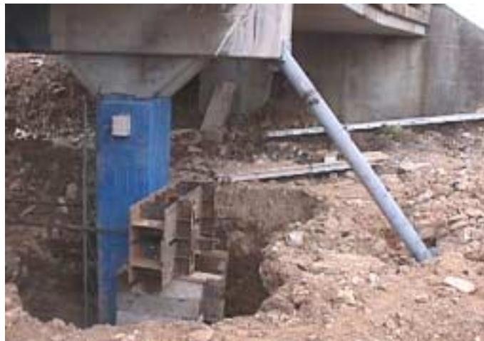
Figure 3.18. Diagonal bracing of the failed column.
