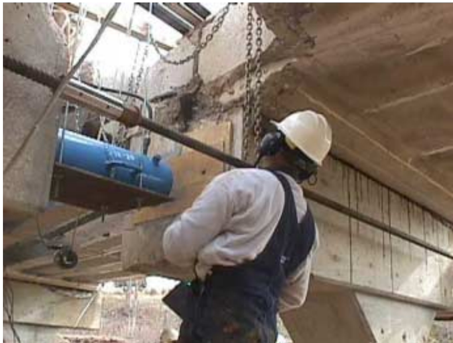
Figure 3.9. Placing the middle jack.
