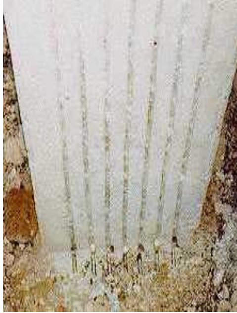
Figure 2.9. Drilled holes at the base of column B2P2 for anchorage of CFRP rods.
