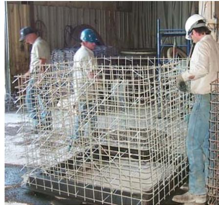
**Figure 3.** GFRP cage
