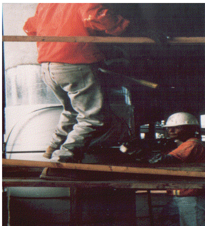
Figure 2a) Clamping the Pre-Fabricated Shell
