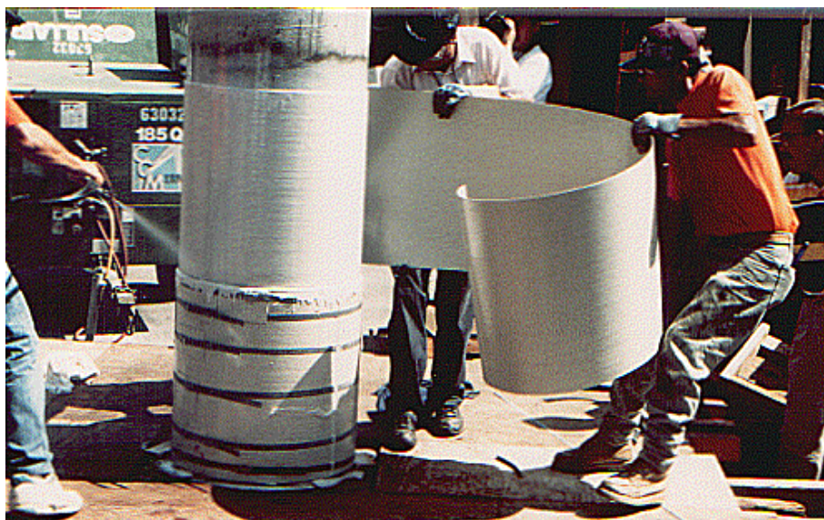
Figure 1 Installing Prefabricated Fiberglass Shell
