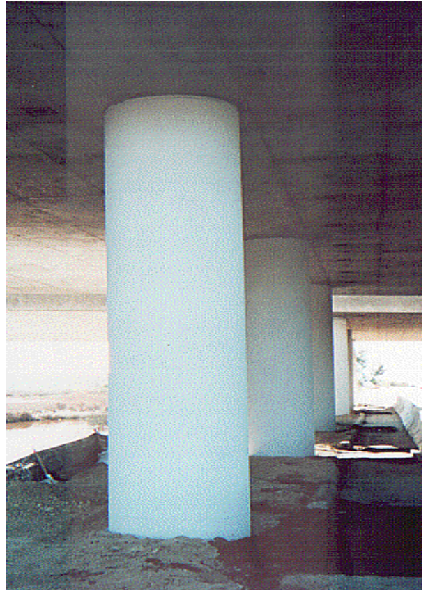
Figure 6 Completed Carbon Fiber Wrap
