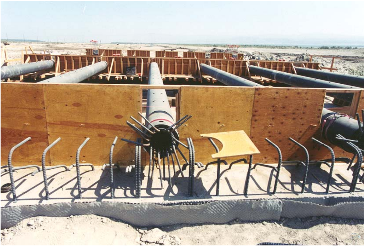
Figure 14 Abutment/Beam Connection
