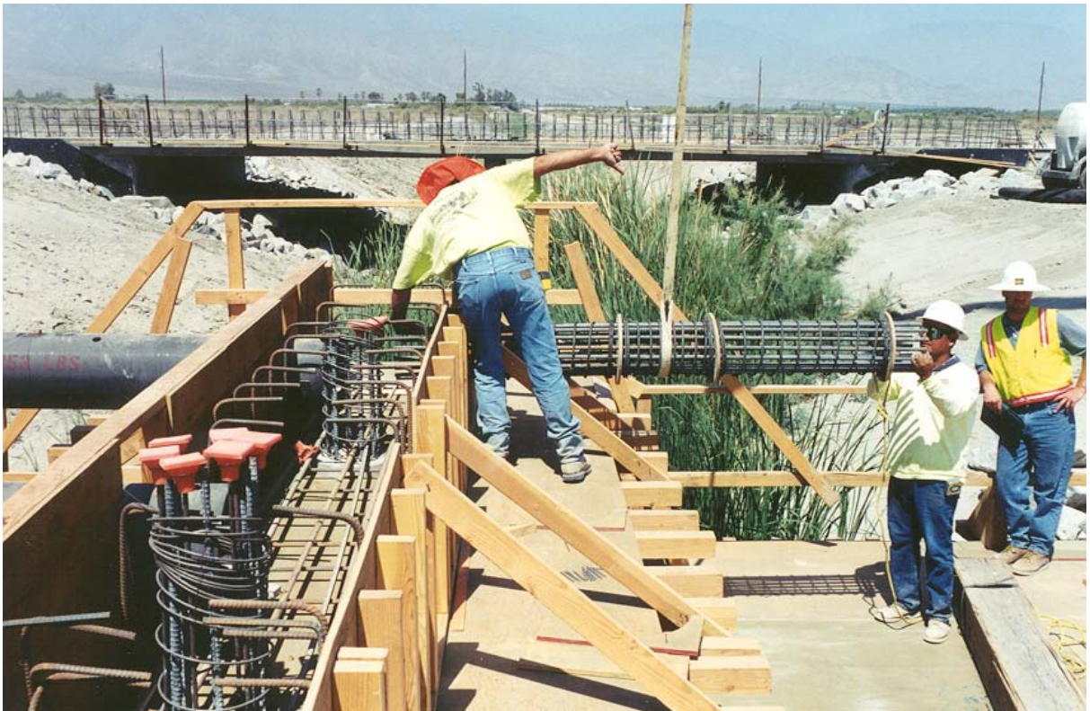
Figure 13 Beam Cap/Girder Connection
