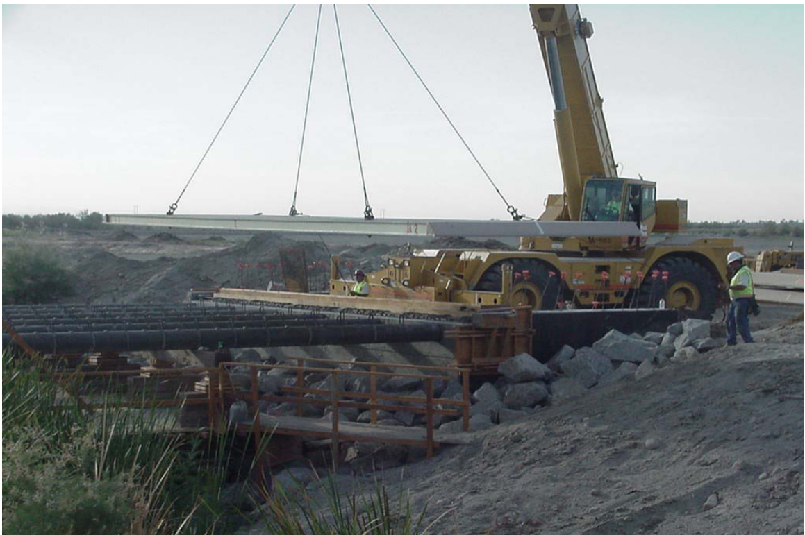
Figure 15 Light Equipment Placing Deck Panel
