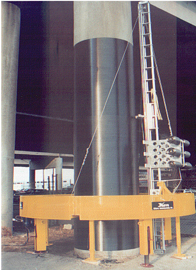
Figure 5 Application of Carbon Fiber ColumnWrap
