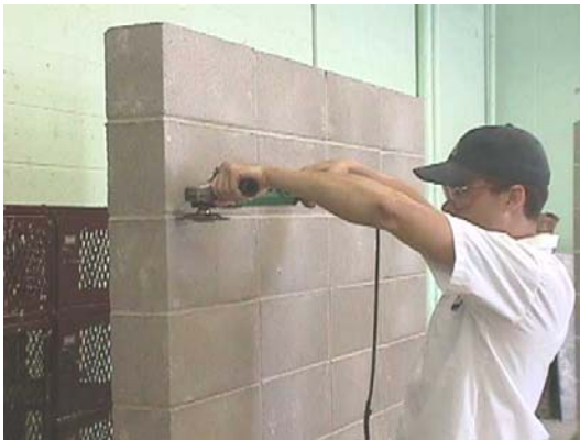
(a) Grinding of Joints
