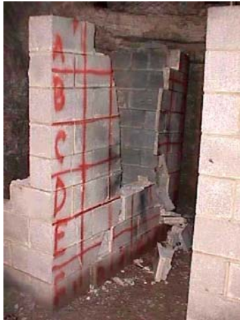
(a) Exterior Face
