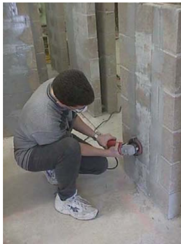
(a) Leveling of Surface
