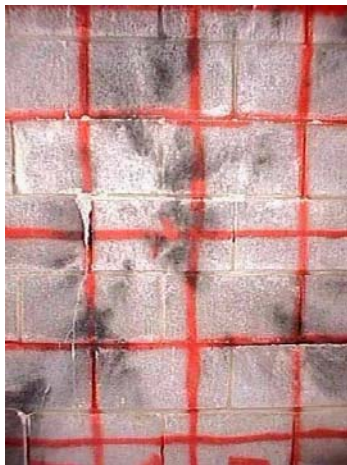
(a) Exterior Face
