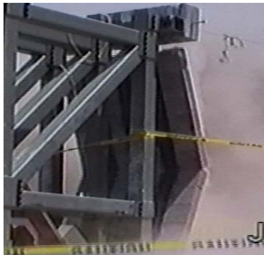
(a) Wall B1 during the Explosion
