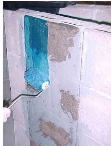
(b) First coat of Saturant
