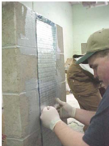
(c) Installation of Fibers
