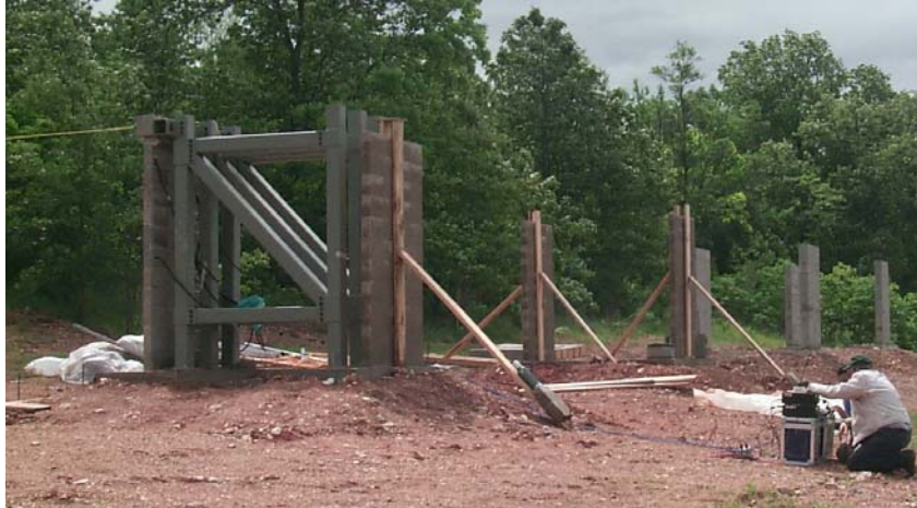
Figure 4.5 The Eight Walls Constructed and Prepared for Testing
