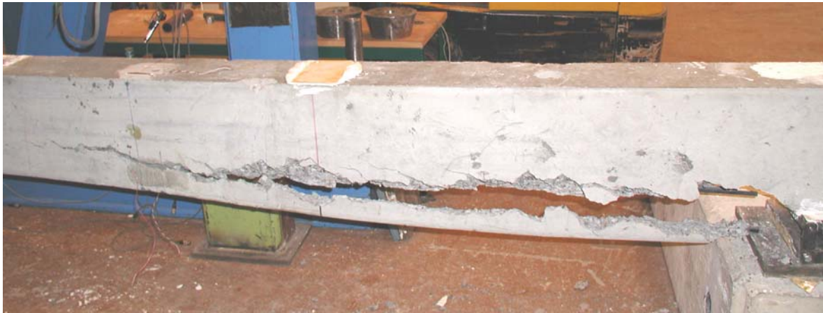
Figure 9. Anchorage failure in the concrete for BM-stat .
