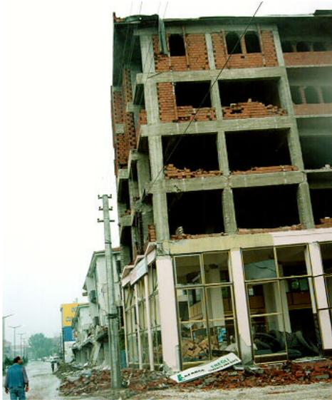
**Figure – 1.** Out-of-Plane Failure – Turkey (1999)
