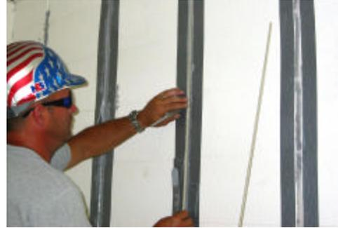
Figure – 9. Installation of GFRP Bar
