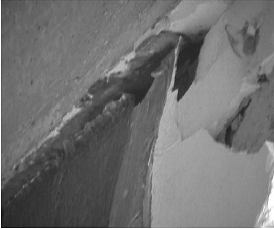
(a) Plaster Delamination (Wall SP)
