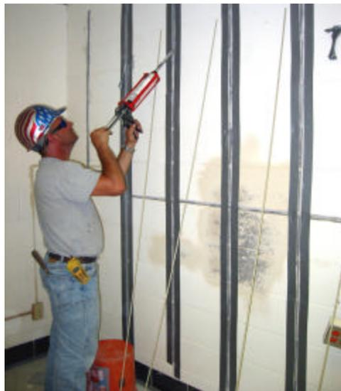
Figure – 8. Application of Epoxy Paste
