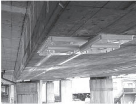
Photograph 2—Applied tensioned CFRP strip
