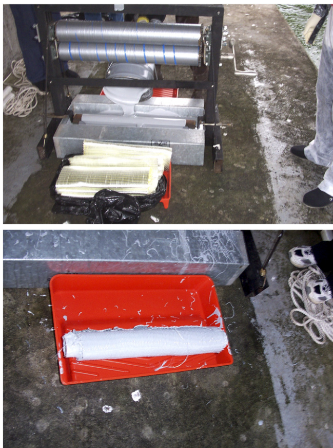
Fig. 8. On-site saturation of fiberglass fabric.
