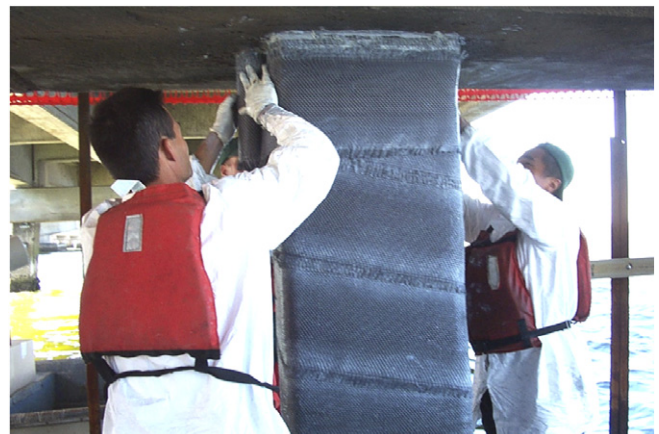
Fig. 7. Applying second transverse CFRP layer.
