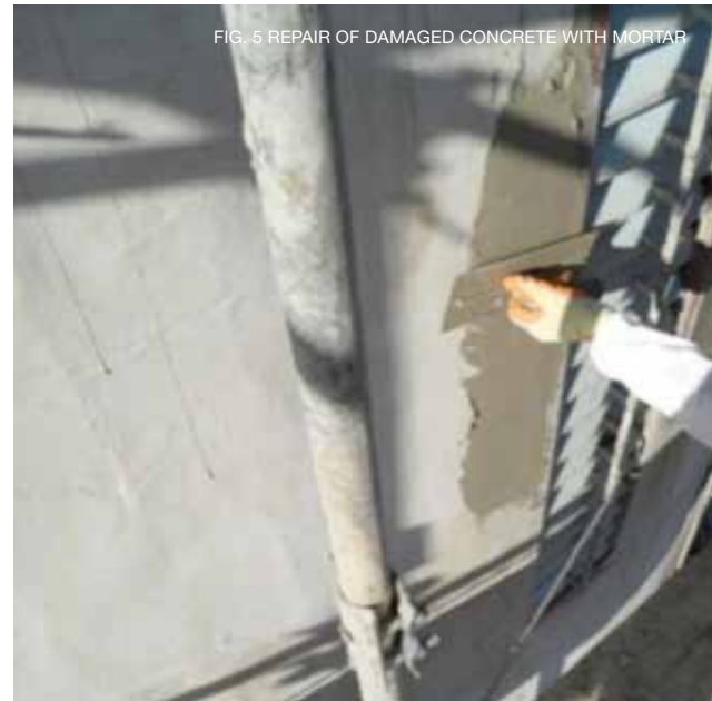
FIG. 6 PATCHING OF DETERIORATED CONCRETE WITH MORTAR
