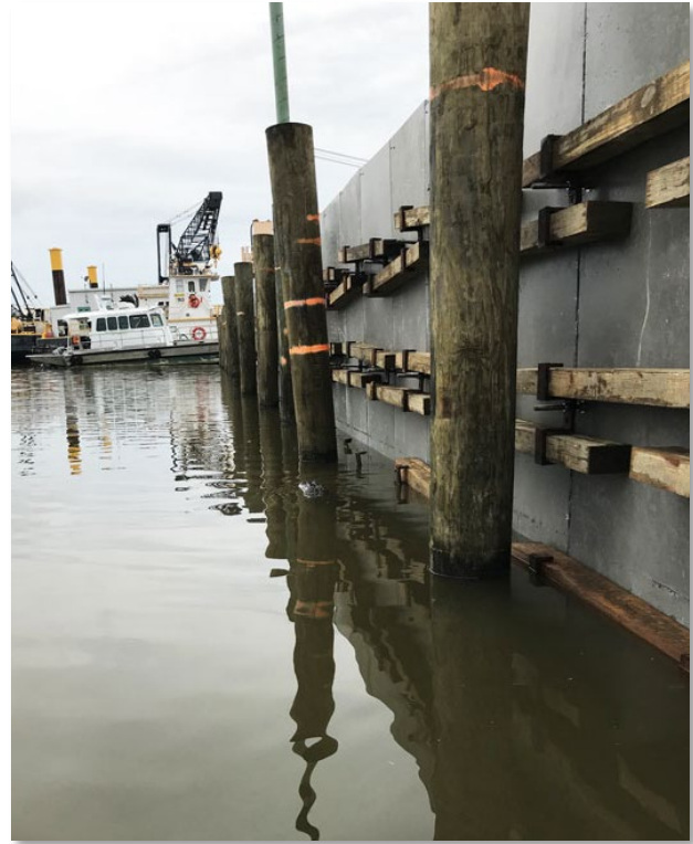
At left, fiberglass rebar cages provide extra strength for non-shrink grout; above, temporary timber walers are put in place while non-shrink grout cures completely.
