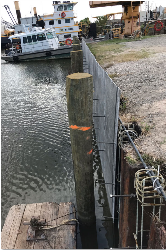
At left, fiberglass rebar cages provide extra strength for non-shrink grout; above, temporary timber walers are put in place while non-shrink grout cures completely.
