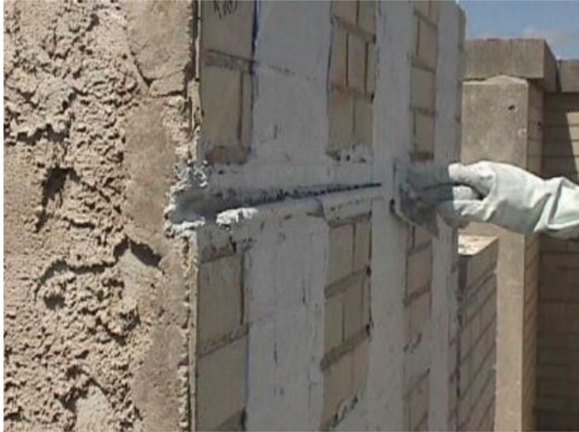
**Figure 1.8. Installation of NSM FRP Rods on Masonry Walls
