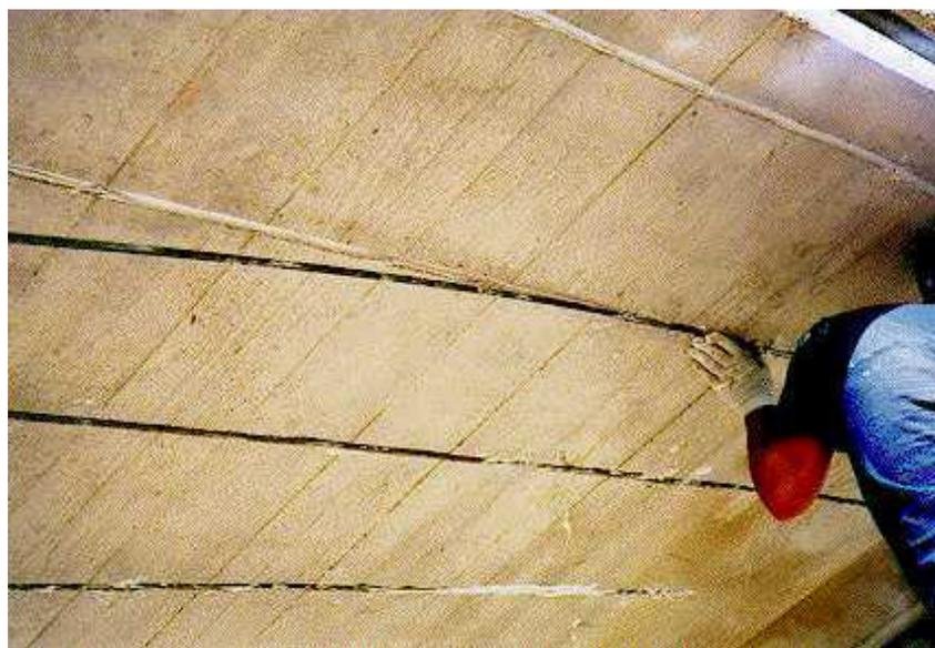
**Figure 1.6. Installation of NSM CFRP Rods in the Bridge Deck (Alkhrdaji et al., 1999)**
