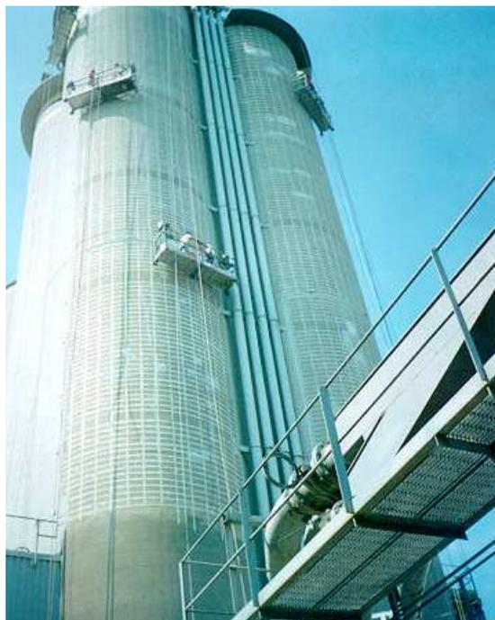
**Figure 1.4. Filling of Grooves with Epoxy Paste (Nanni, 1998)**
