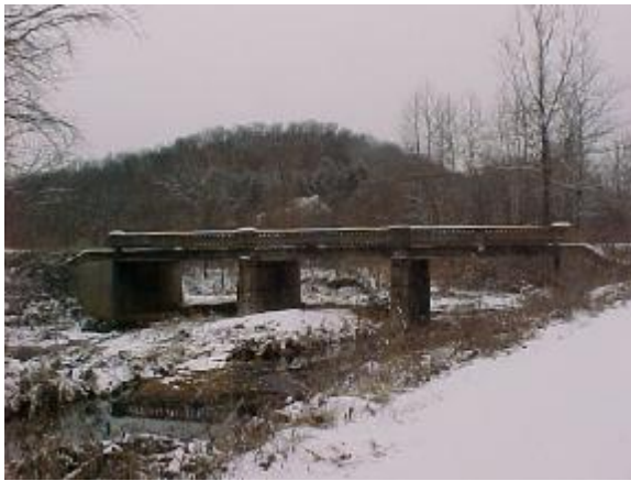
a) Side-view of the Bridge
