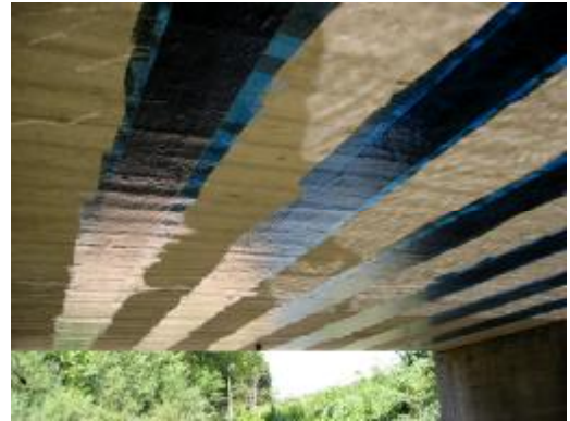
d) Application Completed
