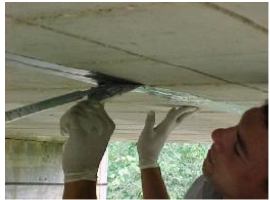
b) Inserting Epoxy Paste into the Groove
