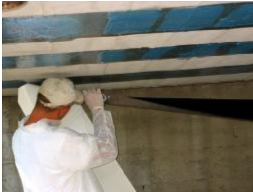
c) Application of CFRP Laminates
