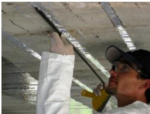
c) Insertion of NSM Bar into the Groove
