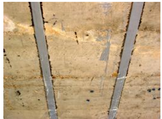
d) Application Completed
