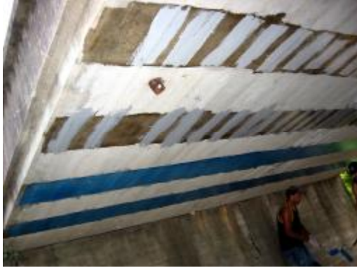
a) Surface Preparation with Primer and Putty
